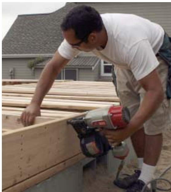
Figure 2. Although balance isn't much of an issue when you're nailing straight down, it's an important consideration in all other framing positions. Max's gun is comfortable to use at any angle, but some of the guns are nose-heavy.
