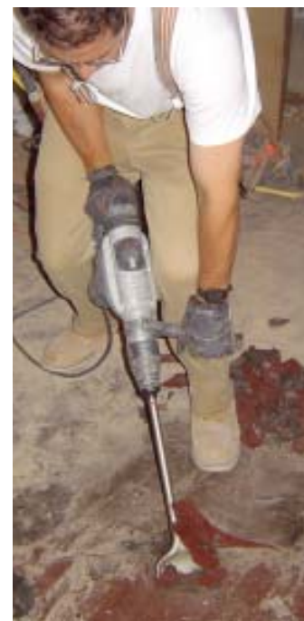
Figure 4. Combination hammers are designed mainly for drilling, but the chipping function comes in handy for a variety of tasks. In the examples shown here, the author breaks out a curb to run a drain into the gutter (left) and, with a wide flat chisel, scrapes up floor tile (right).
