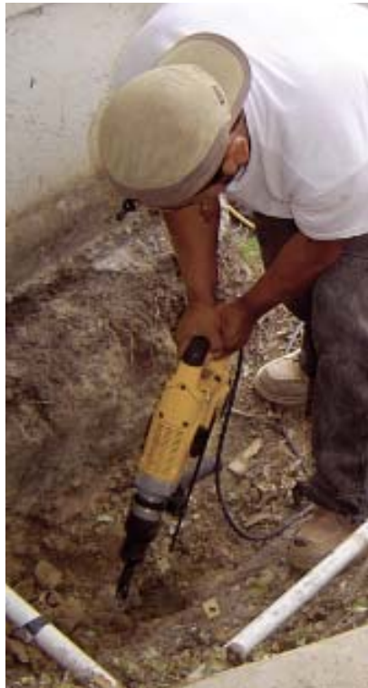
Figure 3. A clay spade (left) is indispensable for loosening packed soil, especially in cramped quarters. Here, a carpenter uses a combination hammer with a clay spade to help dig a trench (right).
