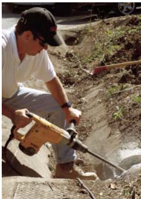
Figure 4. Combination hammers are designed mainly for drilling, but the chipping function comes in handy for a variety of tasks. In the examples shown here, the author breaks out a curb to run a drain into the gutter (left) and, with a wide flat chisel, scrapes up floor tile (right).
