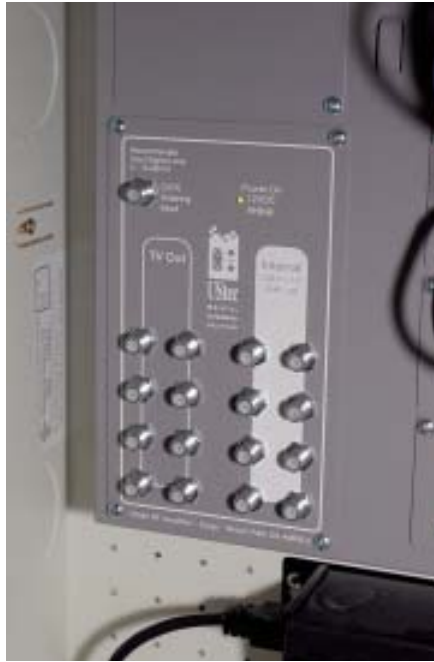
Figure 2. The module with the coaxial connectors on it is a splitter for distributing audio/video signals (right). The blank plates represent open spaces where other modules could be installed. Here (far right), the installer plugs a Cat-5e cable into a module that networks computers.
