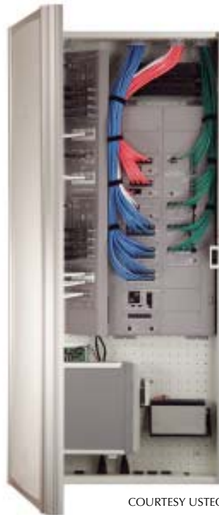
Figure 1. Structured wiring requires many cables, because each one goes directly from the distribution panel to a single receptacle or device. The cables in this panel (left) have been trimmed to length and terminated with RJ-45 and coaxial connectors. When the installation is complete, the panel will resemble the one in this manufacturer's photo (below).
