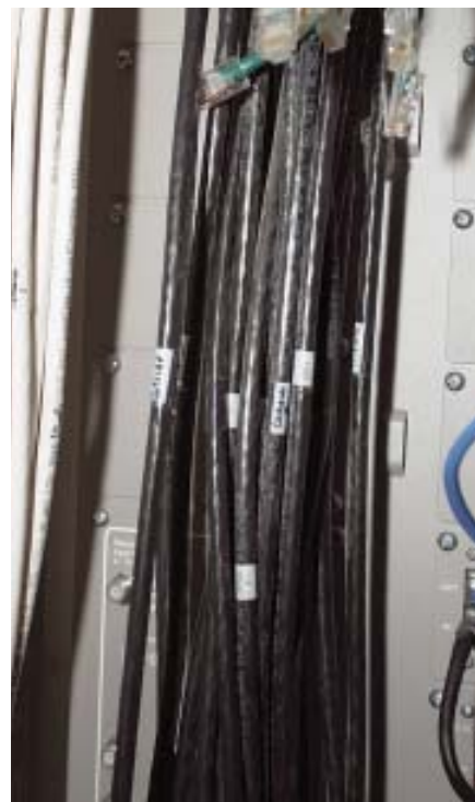
Figure 9. With home-run wiring, there are a lot of cables, so after installation it's important to mark each one with the same information that's on the wiring chart.
