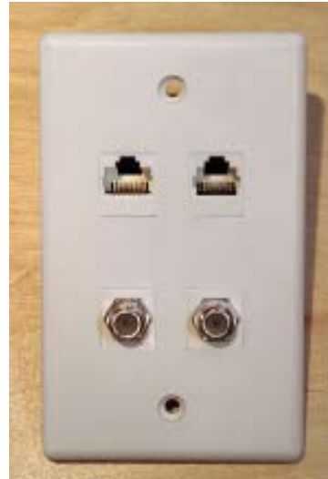
Figure 5. Low-voltage wiring does not require conventional electrical boxes. This green bundled cable goes to a mud ring (left), but it could also go to an open-back box. The cable, which contains two Cat-5e and two coax cables, will terminate at a wall plate (above) with connection points for multiple devices.
