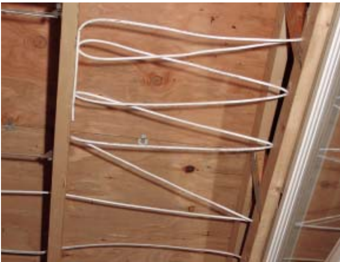
Figure 7. The best way to prewire for future speakers is to leave extra wire and loosely staple it in a zig-zag pattern across the bay. This makes it much easier to find the wire later on.
