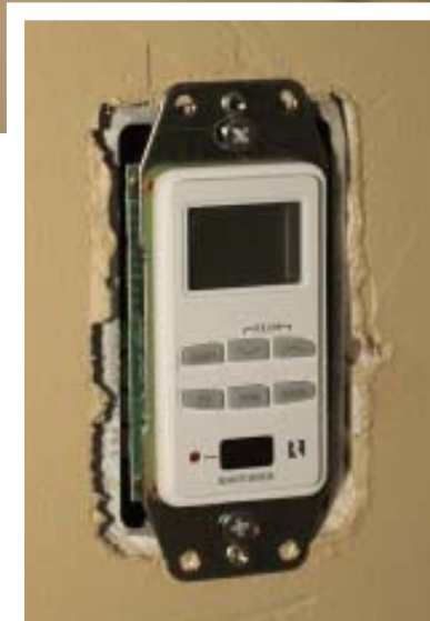
Figure 8. Four twisted pairs of Cat-5e cable clip into the back of a wall-mounted control device (above). Once installed, the device will control the speaker volume in the room and access an audio system that is installed elsewhere in the house (left).
