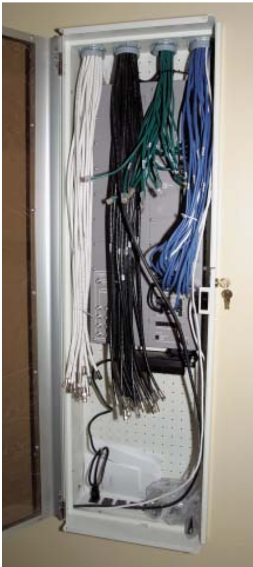
Figure 1. Structured wiring requires many cables, because each one goes directly from the distribution panel to a single receptacle or device. The cables in this panel (left) have been trimmed to length and terminated with RJ-45 and coaxial connectors. When the installation is complete, the panel will resemble the one in this manufacturer's photo (below).
