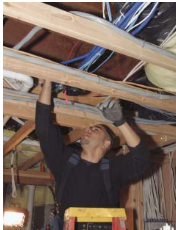
Figure 6. Because household electrical wiring produces interference, the installers keep the blue low-voltage cables away by running them along a different ceiling joist than the Romex (left). If structured wiring has to cross high-voltage wiring, the two types of wire should cross at a 90-degree angle to minimize interference (right). In this case, the low-voltage cables above the joists are perpendicular to the household electrical wire that runs along the sides.
