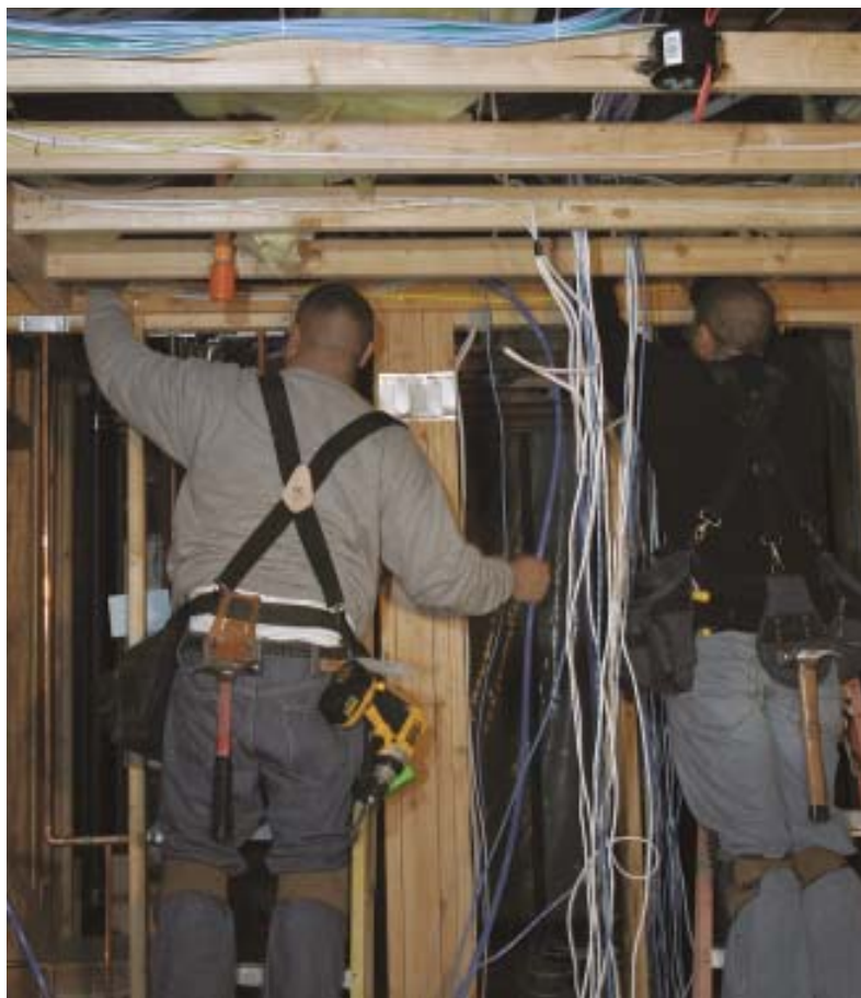
Figure 6. Because household electrical wiring produces interference, the installers keep the blue low-voltage cables away by running them along a different ceiling joist than the Romex (left). If structured wiring has to cross high-voltage wiring, the two types of wire should cross at a 90-degree angle to minimize interference (right). In this case, the low-voltage cables above the joists are perpendicular to the household electrical wire that runs along the sides.
