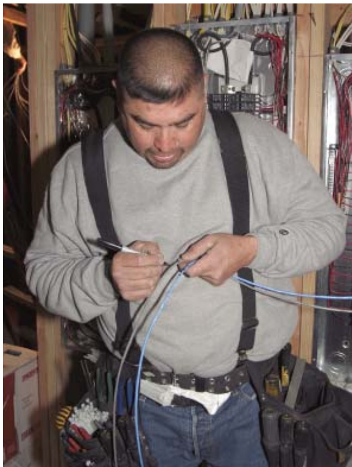
Figure 9. With home-run wiring, there are a lot of cables, so after installation it's important to mark each one with the same information that's on the wiring chart.
