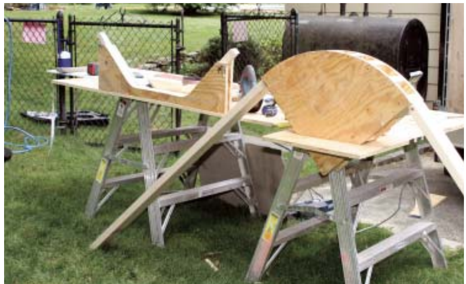
Figure 1. After laying out the 20-inch radius of the outside corners of the pool deck, a crew member built a form out of plywood and framing lumber with the same radius (above); this form would be used to mold the outside skirtboard. For the inside corners, a tracing was made of the pool's coping, and then a plywood form was built to match (above right).
