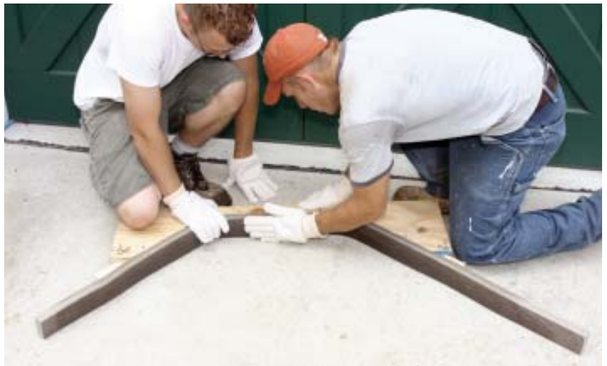
Figure 4. Ripped to a thinner width to fit on top of the pool's coping, the inner skirts were extremely flexible after heating (top) and conformed to the angular shape of the form with only hand pressure (above). The right temperature is critical when molding complex shapes: If it gets too hot, Trex deforms, but if it's not hot enough, it can tear (left).
