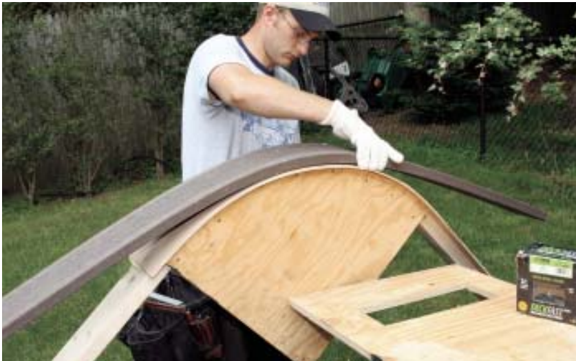
Figure 3. When placed on the radiused form, the heat-treated Trex board easily relaxed into shape (above). A crew member lightly clamped the board ends to coax them the last couple of inches into their final position (right), then allowed the board to cool.
