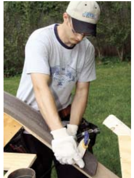
Figure 3. When placed on the radiused form, the heat-treated Trex board easily relaxed into shape (above). A crew member lightly clamped the board ends to coax them the last couple of inches into their final position (right), then allowed the board to cool.
