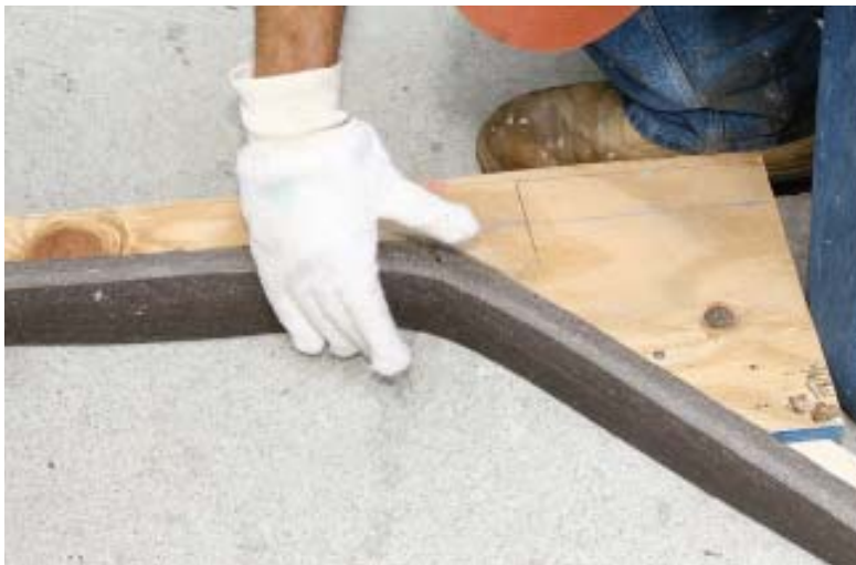
Figure 4. Ripped to a thinner width to fit on top of the pool's coping, the inner skirts were extremely flexible after heating (top) and conformed to the angular shape of the form with only hand pressure (above). The right temperature is critical when molding complex shapes: If it gets too hot, Trex deforms, but if it's not hot enough, it can tear (left).
