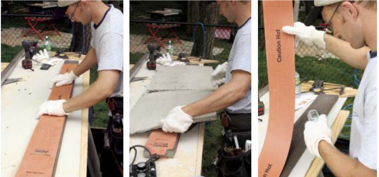
Figure 2. To heat the Trex enough to mold it to the shape of the forms, the author's crew used temperature-regulated Heatcon heating blankets (left). Sandwiching the Trex between sheets of scrap cement backerboard and fireproof Sheetrock helped minimize external heat loss and speed up the heating process (center). A few degrees makes a big difference in the workability of the board; the infrared thermometer included in the Heatcon kit allowed the crew to track the surface temperature accurately (right).
