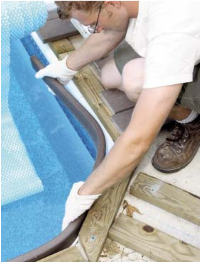
Figure 5. As with the outside corners, the inside corner skirts were installed first, with stainless fasteners screwed into the sleepers, followed by the remaining sections of skirt (above). In the completed project, the top of each skirt is flush with the surface of the decking (right).
