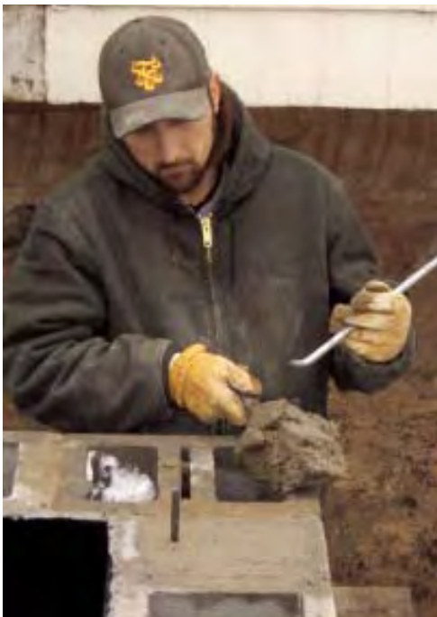
Figure 12. The anchor bolts were set into grout-filled cores so that only 3 inches were left exposed (left). Then the bolt holes were counterbored to accept the nuts and washers (above).
