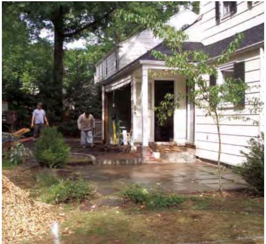
Figure 1. The spray-painted lines represent the approximate outside edge of the addition's footing; the excavator dug 3 feet beyond them to allow room for laying the foundation drain, parging, and dampproofing. Woodchips were used to cushion the impact of the excavator on a nearby tree's root system.
