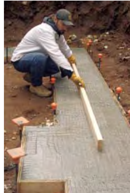
Figure 3. Placed in an 8-inch-deep trench dug into the bottom of the excavation (left), the footings were reinforced with parallel lengths of \frac{1}{2} -inch rebar wired together and held off the ground and away from the form edges by chairs (center). For safety, the author's crew makes it standard practice to cap exposed stakes and rebar (right).
