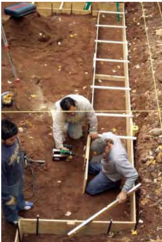
Figure 3. Placed in an 8-inch-deep trench dug into the bottom of the excavation (left), the footings were reinforced with parallel lengths of \frac{1}{2} -inch rebar wired together and held off the ground and away from the form edges by chairs (center). For safety, the author's crew makes it standard practice to cap exposed stakes and rebar (right).
