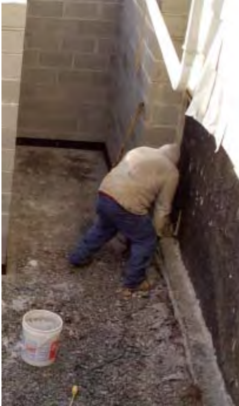
Figure 10. Before pouring the basement slab, workers attached lengths of expansion joint filler to the interior perimeter of the block wall (left), then laid down a 6-mil poly vapor barrier and wire mesh (below). Sheets of plywood and plastic protected the walls from splashing concrete (bottom).
