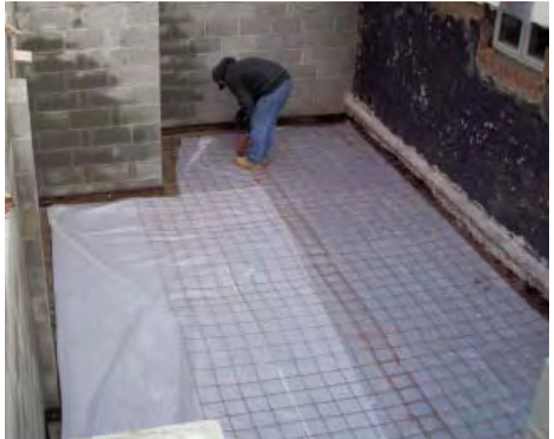
Figure 10. Before pouring the basement slab, workers attached lengths of expansion joint filler to the interior perimeter of the block wall (left), then laid down a 6-mil poly vapor barrier and wire mesh (below). Sheets of plywood and plastic protected the walls from splashing concrete (bottom).
