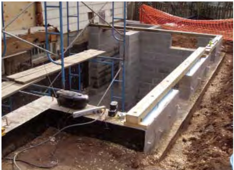
Figure 12. The anchor bolts were set into grout-filled cores so that only 3 inches were left exposed (left). Then the bolt holes were counterbored to accept the nuts and washers (above).
