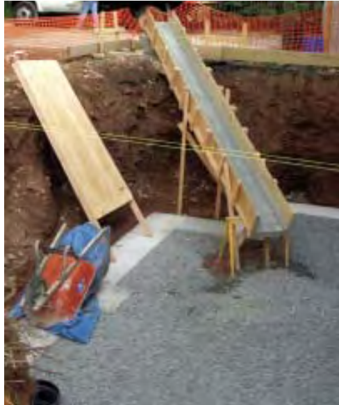
Figure 4. A plywood chute made it easier to place concrete for the footings (far left). Later, the chute was used to slide stone (left) and block into the hole, and to pour the basement slab.
