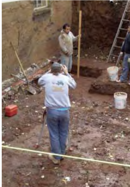
Figure 2. After excavation, the author's crew dug the 8-inch-deep footing trench by hand, using the top of the existing footing as a benchmark.
