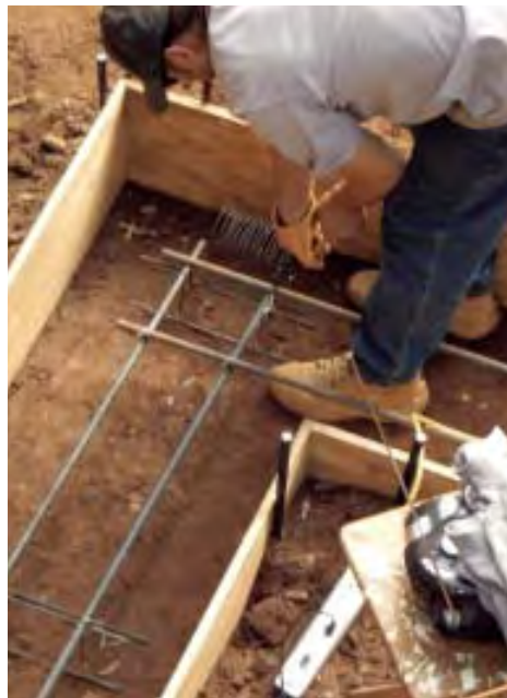
Figure 3. Placed in an 8-inch-deep trench dug into the bottom of the excavation (left), the footings were reinforced with parallel lengths of \frac{1}{2} -inch rebar wired together and held off the ground and away from the form edges by chairs (center). For safety, the author's crew makes it standard practice to cap exposed stakes and rebar (right).
