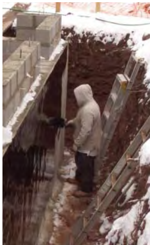
Figure 9. Parging — applying a ½-inch-thick layer of mortar with a trowel and screeding it smooth with a straight-edge — helped seal the porous surface of the concrete-block foundation (right), while a brushed-on coat of cold asphalt (far right) damp-proofed the wall.
