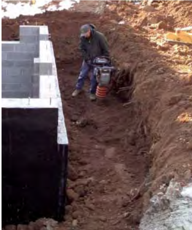
Figure 11. The wall was backfilled and hand-compacted in 2-foot lifts to avoid putting too much lateral pressure on the foundation.
