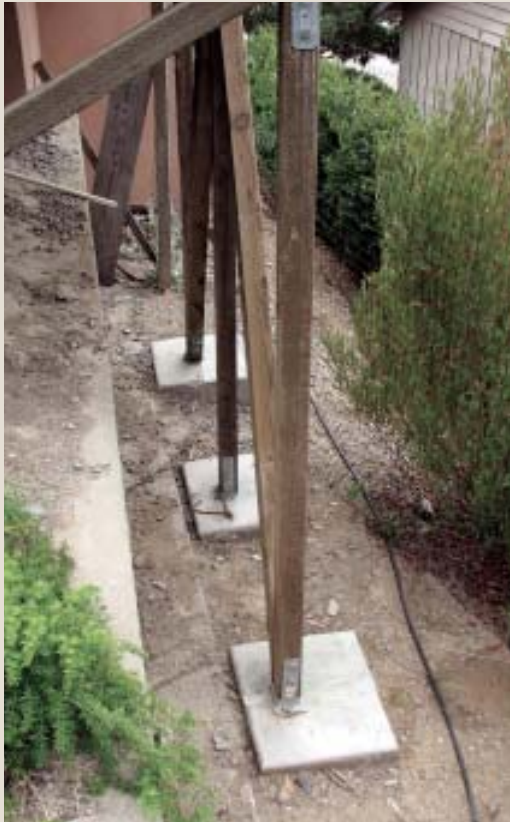
Figure 4. The author cross-braced the end of the deck with 4x6 diagonals (above), which he fastened to the corner posts with the same bolts that hold the posts in the column bases (above right). The diagonals butt to a post at midspan and are bolted to it through the same Simpson CC44 column cap that connects the post to the beam above (right).
