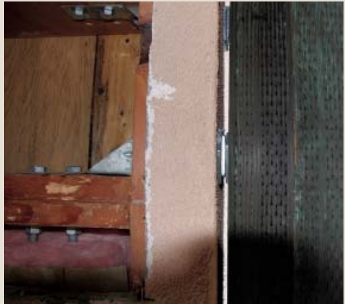
Figure 2. Since a continuous glass handrail will prevent water from draining off the outer edge of the deck, the author sloped the joists toward the house (above left) and used stacks of 3-inch-square washers to space the ledger beam off the wall (above right). Water drains through this space and is collected by a gutter below the deck (left).
