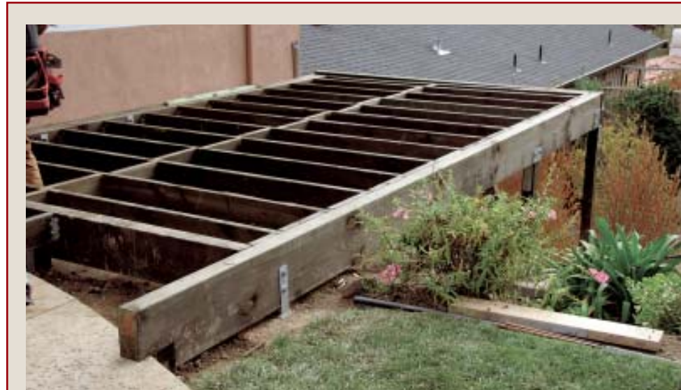
Figure 1. The joists run between a 4x10 ledger beam and a 4x12 outer beam carried by posts on concrete piers (above). One end of the deck laps about 5 feet onto an existing concrete patio (left and opposite).
