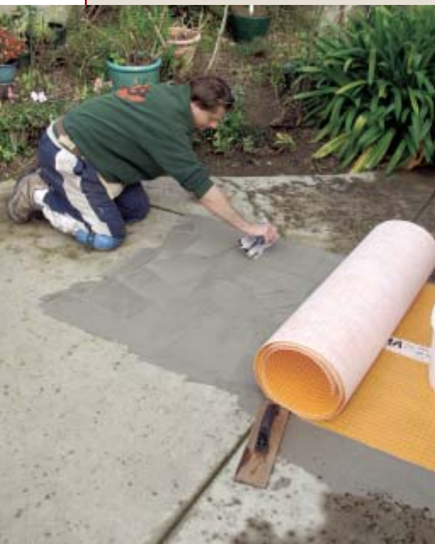
Figure 6. To accommodate possible movement in the slab, the tile contractor installed an isolation membrane, applying unmodified thinset to the substrate (left) and then pressing the membrane into place with a float (above).
