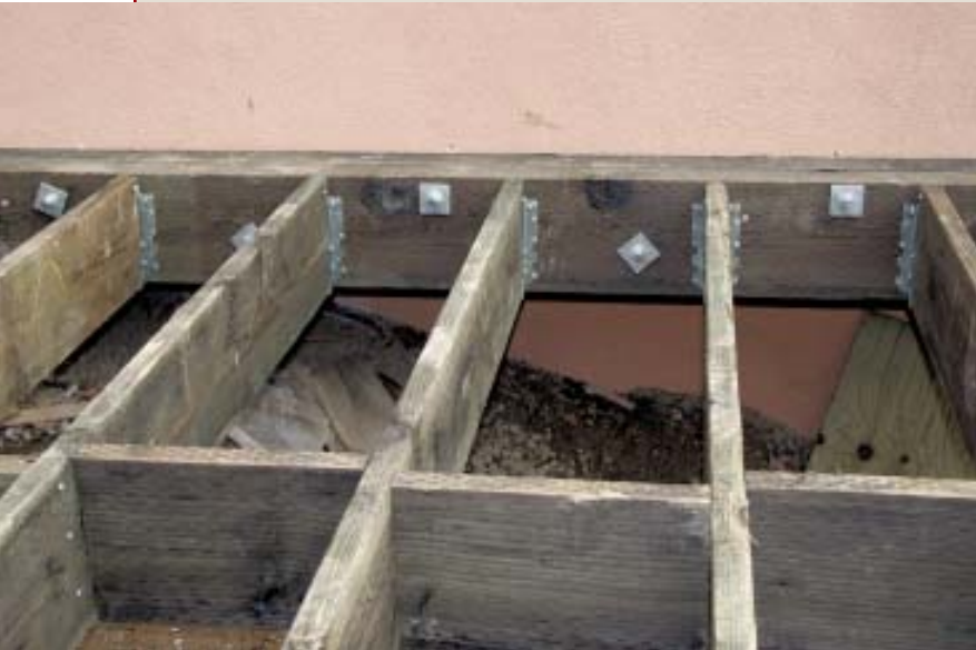
Figure 3. The left end of the ledger beam (above) is bolted to the house with \frac{5}{8} -inch all-thread that runs between nuts and washers outside and Simpson HD2A hold-downs inside (above right). This ties the ledger to the joists instead of to the rim — which, because the joists are cantilevered, is not supported by a sill.
