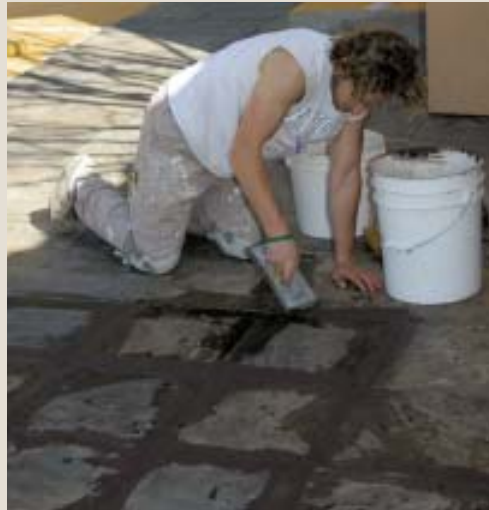
Figure 8. The tile was set in unmodified thin-set (far left), then grouted (left). The completed job adds an outdoor room to the house (below).
