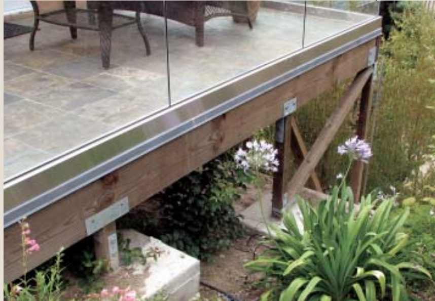
Figure 5. After the cement board was installed, the glazing contractor bolted the aluminum base shoe (above left) over a galvanized flashing at the edge of the deck (left). Later, when the tile had been set, he cemented 1/2-inch tempered-glass panels into the channel, then clad the channel with a stainless steel cover (above).
