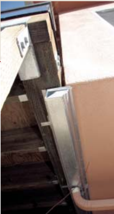
Figure 2. Since a continuous glass handrail will prevent water from draining off the outer edge of the deck, the author sloped the joists toward the house (above left) and used stacks of 3-inch-square washers to space the ledger beam off the wall (above right). Water drains through this space and is collected by a gutter below the deck (left).
