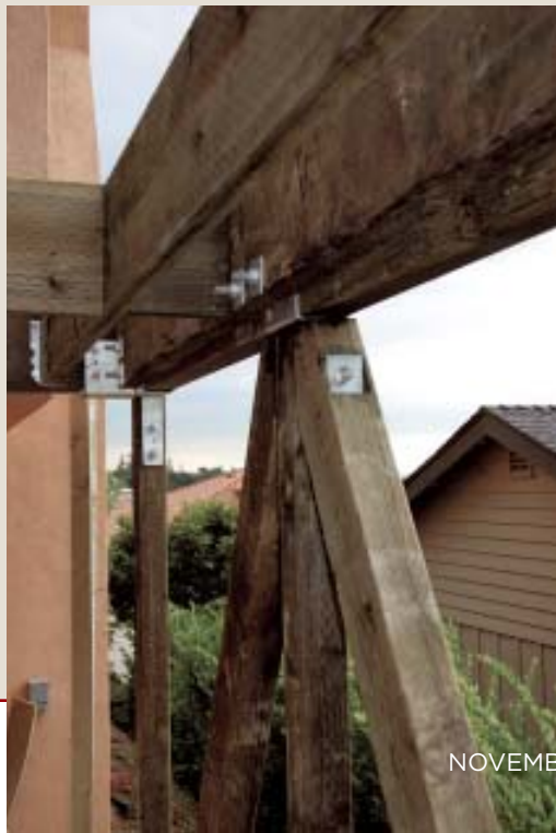
Figure 4. The author cross-braced the end of the deck with 4x6 diagonals (above), which he fastened to the corner posts with the same bolts that hold the posts in the column bases (above right). The diagonals butt to a post at midspan and are bolted to it through the same Simpson CC44 column cap that connects the post to the beam above (right).
