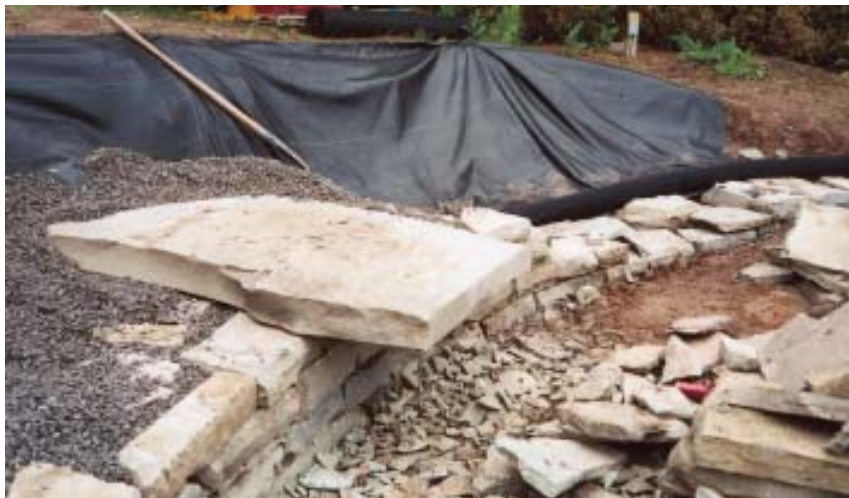
Figure 5. Three 6-foot-long stone slabs were cantilevered about 18 inches out from the wall at roughly 18 inches above finished grade to create informal seating. The weight of the stones, the backfill material, and the wall above the slabs will help hold them securely in place.
