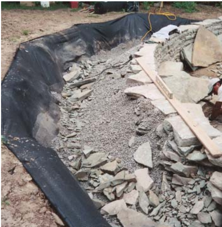
Figure 7. Resembling a triangle in cross section, the retaining wall is carefully backfilled with unusable stone, rubble from cuts, and crushed stone. Members of the author's crew rely on spirit levels and a trained eye to ensure that the curved wall remains both level and consistently battered back about 10 degrees from the vertical while they lay up stone.
