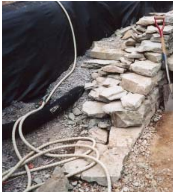
Figure 3. A stable, well-drained base of crushed stone will help prevent the wall from settling, and minimize damage from freeze/thaw cycles. A 4-inch perforated daylight drainpipe has been placed at the base of the wall; it's shown here wrapped in fabric and covered with stone.
