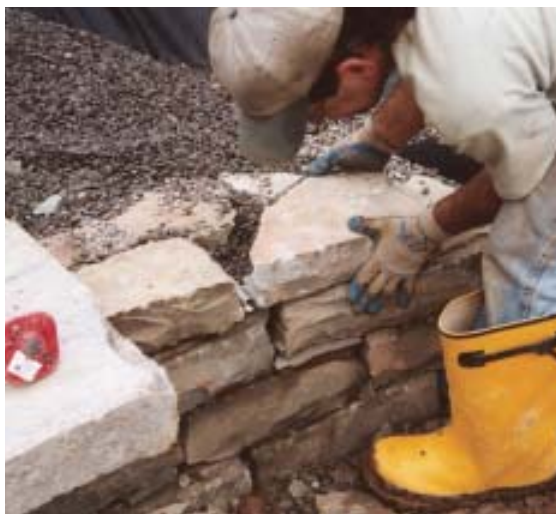
Figure 6. When placing the stones, it's best to avoid vertical joints and try to overlap each stone over two others. Here, the worker had to align two joints to make room for electrical conduit that will eventually supply built-in lighting fixtures.
