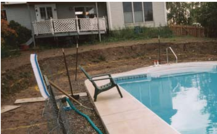
Figure 1. The first step in constructing any kind of stone wall is verifying that disturbed soils have completely settled; only then should rough grading and layout begin. Here, the yellow line painted on the ground indicates the approximate position of the new wall.
