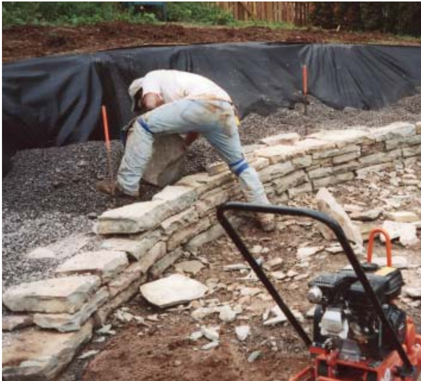
Figure 4. To reduce soil pressure, the ground has been excavated behind the retaining wall at an angle of about 45 degrees, then backfilled with #2 crushed stone to enhance drainage. Lining the excavation with landscape fabric helps keep soil from washing into the crushed stone, which would diminish its ability to drain properly.
