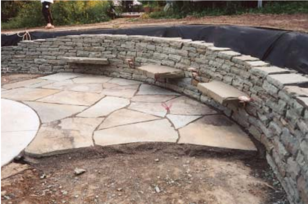
Figure 8. Flat, smooth coping stones cap the retaining wall. Mushroom-shaped low-voltage lighting fixtures mounted in the wall beside the stone benches provide illumination for the poolside sitting area.
