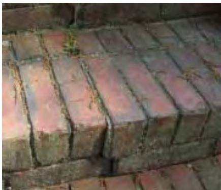
Figure 1. Laid directly on soil (top), the bricks of this 65-year-old staircase were displaced by as much as an inch in some areas (above). The mixture of large, unyielding rocks and soft, loamy clay underlying the steps caused the differential movement (right).
