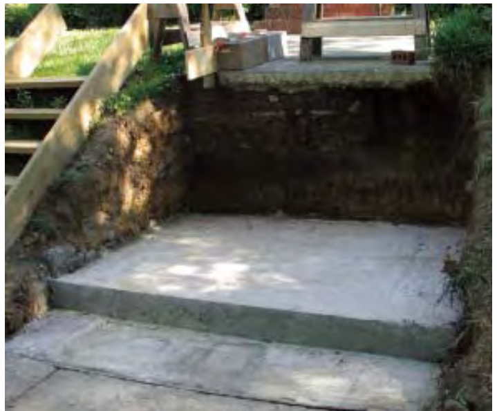
Figure 2. To provide a solid base for the stair's concrete footing, the author had to remove or break apart large rocks and excavate down to firm soil (above). The finished footing (right) steps up exactly the height of one brick step and is pitched about \frac{1}{4} inch per foot for drainage.
