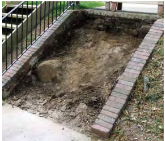
Figure 1. Laid directly on soil (top), the bricks of this 65-year-old staircase were displaced by as much as an inch in some areas (above). The mixture of large, unyielding rocks and soft, loamy clay underlying the steps caused the differential movement (right).
