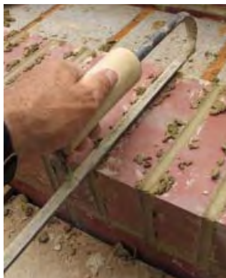
Figure 7. With a sled jointer, the author packed the mortar tight and made clean, concave, water-resistant joints.
