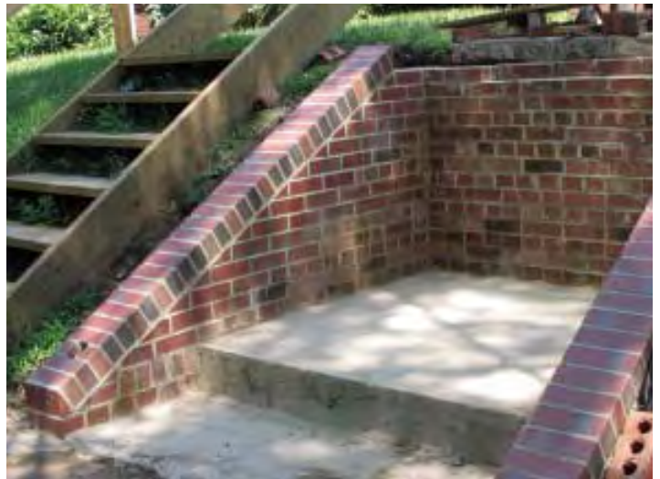
Figure 3. Brackets built with scrap 2-by material held the strings the author used for setting the field brick for the wing walls (left) and the rowlock border (below left). Because bricks with full mortar joints resist water intrusion better than concrete block, the author used brick left over from earlier jobs for the below-grade portions of the walls (below).
