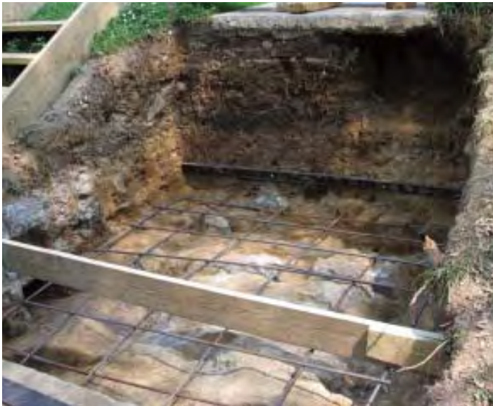
Figure 2. To provide a solid base for the stair's concrete footing, the author had to remove or break apart large rocks and excavate down to firm soil (above). The finished footing (right) steps up exactly the height of one brick step and is pitched about \frac{1}{4} inch per foot for drainage.
