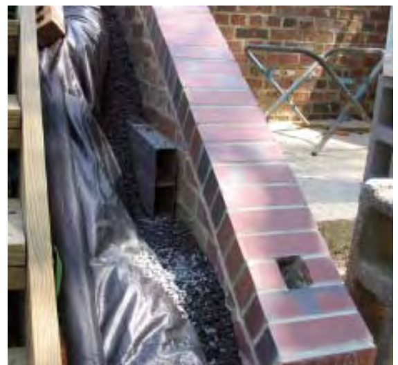
Figure 5. A perimeter drain system around the base of the wing walls helps guide groundwater away from the steps, keeping hydrostatic pressure to a minimum.
