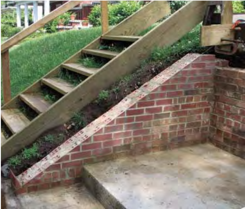
Figure 3. Brackets built with scrap 2-by material held the strings the author used for setting the field brick for the wing walls (left) and the rowlock border (below left). Because bricks with full mortar joints resist water intrusion better than concrete block, the author used brick left over from earlier jobs for the below-grade portions of the walls (below).
