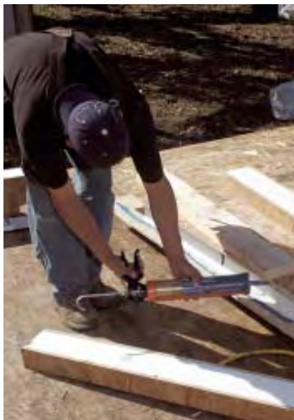
Figure 5. Panels are connected edge-to-edge with splines. Here, a carpenter prepares to install a block spline over continuous beads of sealant (left). The spline functions as a gusset and is held in place with nails driven first into the loose panel (center) and then into the adjoining panel (right).
