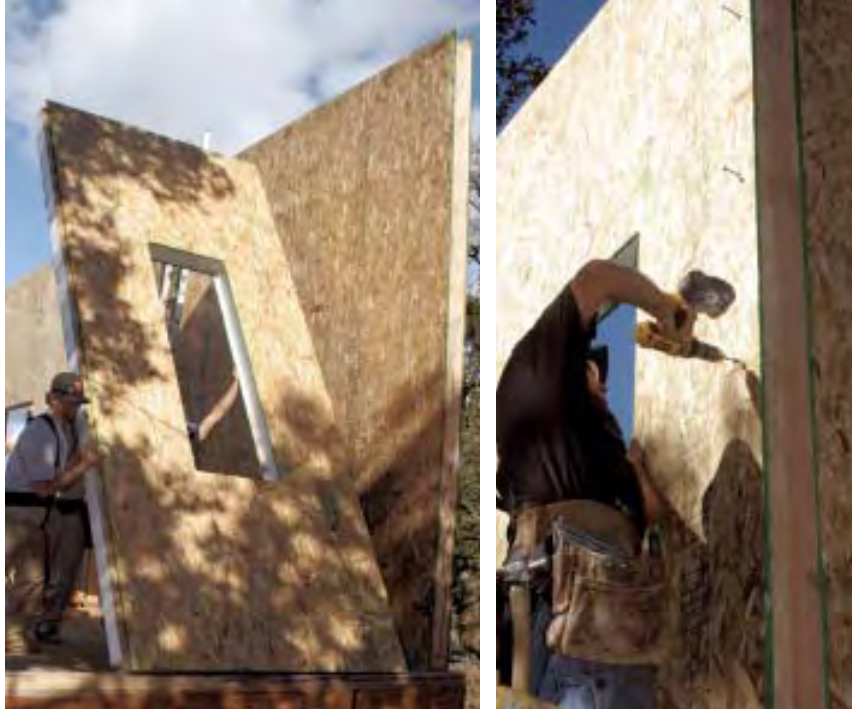
Figure 6. At corners, the crew installs nailers flush to the edge of the panels, butts the panels together (left), and uses screws to fasten through to the nailer beyond (right). These panels are 6½ inches thick, requiring 8-inch-long screws.
