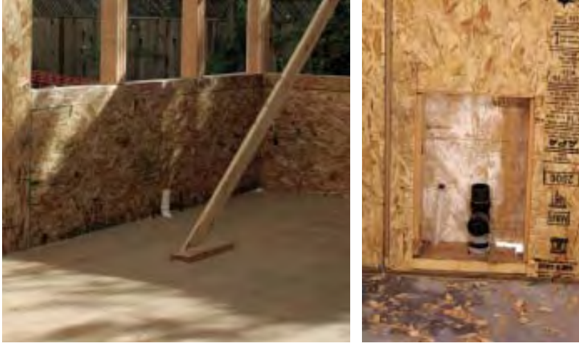
Figure 10. To avoid putting pipes in the wall, the author had the plumber install the drain and supply lines for a sink just inside the panels at the sink-cabinet location (far left). If plumbing must go in an exterior wall, the author creates a chase by cutting out the panel and removing some of the foam (left). Once rough-in is complete, the author's crew uses spray foam to fill in around the pipes.
