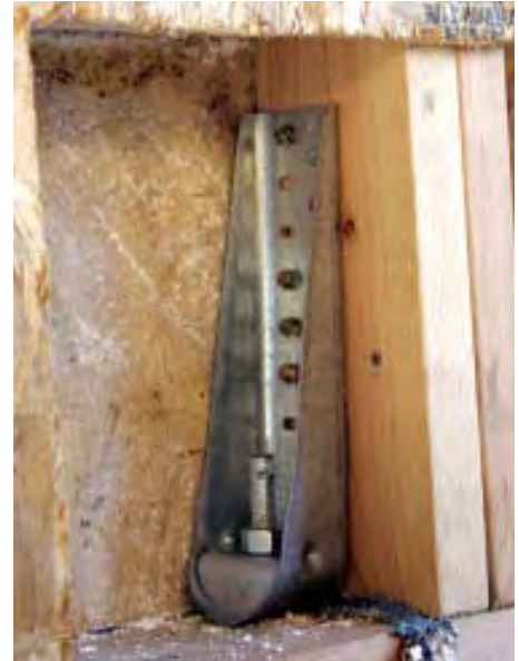
Figure 4. The OSB and foam were cut from the corner of this SIP shear wall so that a hold-down could be installed. Later the crew will foam in around it and replace the missing OSB.
