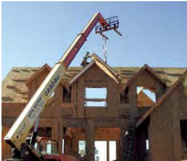
Figure 2. Panels can be used for any part of the building that isn't curved. The walls and roof of this traditional-style house are made from SIPs.
