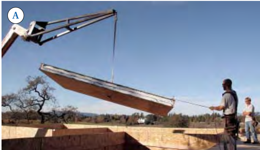
Figure 7. Roof panels are lifted with an all-terrain forklift (A) and lowered onto glulam beams and sloped ledgers screwed to the wall panels (B). This carpenter fastens a panel by screwing through to the beam below (C). The parapets terminate with a double top plate, specified by the engineer (D).
