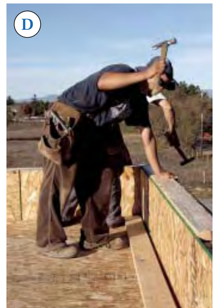
Figure 7. Roof panels are lifted with an all-terrain forklift (A) and lowered onto glulam beams and sloped ledgers screwed to the wall panels (B). This carpenter fastens a panel by screwing through to the beam below (C). The parapets terminate with a double top plate, specified by the engineer (D).
