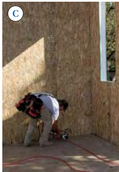
Figure 3. Plates are installed first. Here, a 3x6 has been screwed to the deck over a continuous bead of sealant. In preparation for standing the walls, a carpenter runs sealant along the face and edges of the plate (A). The crew then stands the panel over the plate (B), braces it plumb, and nails it to the sides of the plate (C). When walls land on concrete, the plate is installed over a wider strip of pressure-treated plywood, which is also sealed to the concrete (D).
