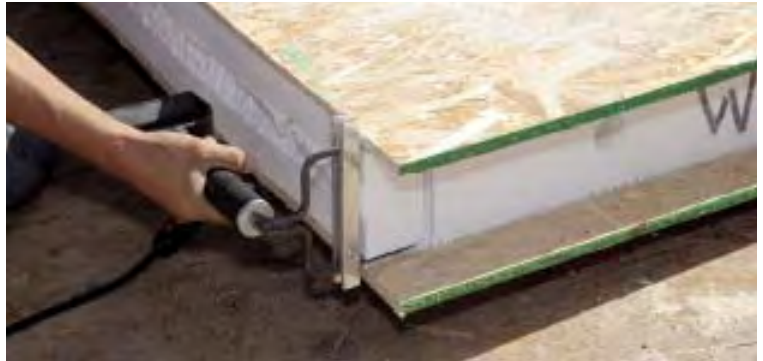
Figure 9. Mistakes and changes sometimes force the crew to alter panels in the field. Here, a carpenter trims a panel to size (left), then uses an electric hot knife (below) to neatly remove the foam so there will be room for a block spline.
