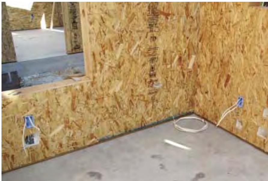
Figure 11. Wire chases are provided by panel manufacturers. The electrician accesses the chase by cutting a hole through the OSB and removing some of the foam. He can then fish wires through the chases and connect them to remodeling boxes in the panels.
