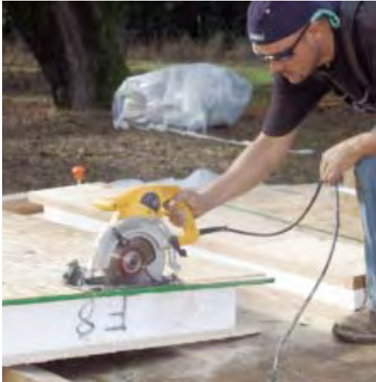
Figure 9. Mistakes and changes sometimes force the crew to alter panels in the field. Here, a carpenter trims a panel to size (left), then uses an electric hot knife (below) to neatly remove the foam so there will be room for a block spline.
