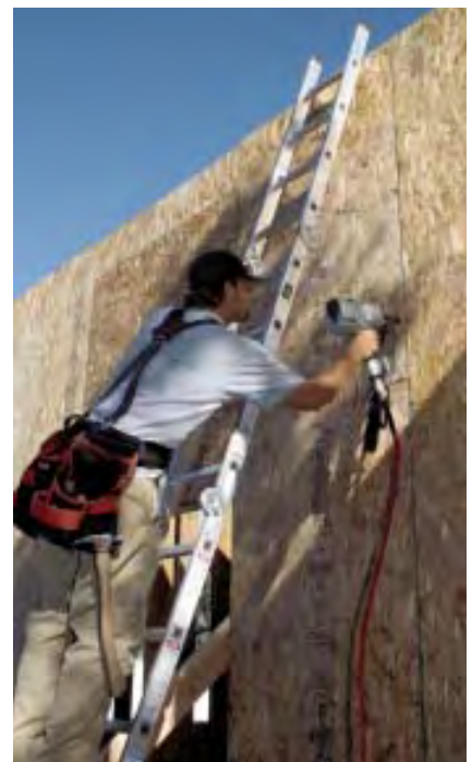
Figure 5. Panels are connected edge-to-edge with splines. Here, a carpenter prepares to install a block spline over continuous beads of sealant (left). The spline functions as a gusset and is held in place with nails driven first into the loose panel (center) and then into the adjoining panel (right).
