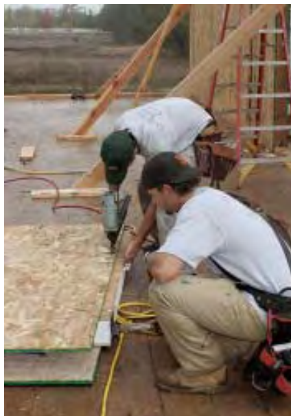
Figure 5. Panels are connected edge-to-edge with splines. Here, a carpenter prepares to install a block spline over continuous beads of sealant (left). The spline functions as a gusset and is held in place with nails driven first into the loose panel (center) and then into the adjoining panel (right).
