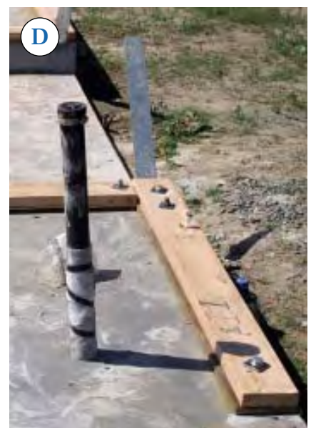
Figure 3. Plates are installed first. Here, a 3x6 has been screwed to the deck over a continuous bead of sealant. In preparation for standing the walls, a carpenter runs sealant along the face and edges of the plate (A). The crew then stands the panel over the plate (B), braces it plumb, and nails it to the sides of the plate (C). When walls land on concrete, the plate is installed over a wider strip of pressure-treated plywood, which is also sealed to the concrete (D).
