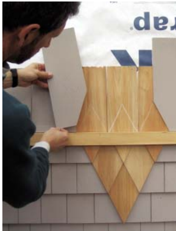
Figure 4. Tapered ramp shingles — thin strips sliced from full shingles — are the key to this layered design (top left). The thickness of the ramp butt matches the butt thickness of the diamond shingle at the course line, allowing adjoining shingles to feather up to meet the pattern. Once the pattern has reached the desired width, the author uses reverse-point shingles (left) to close the diamond, filling in with pointed shingles (above).
