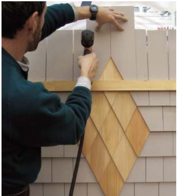
Figure 5. To finish the diamond, the author fastens the final point shingle between a pair of reverse-point shingles (above right), then installs the reverse-point shingles that close the top (right).
