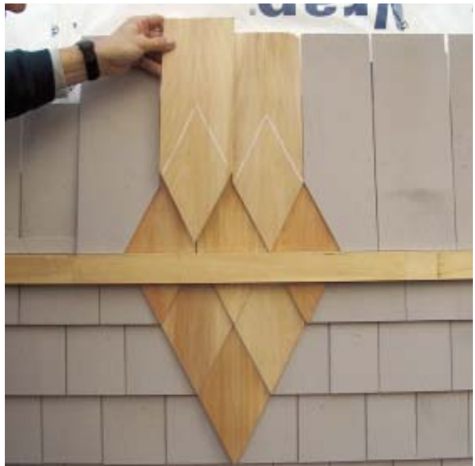
Figure 4. Tapered ramp shingles — thin strips sliced from full shingles — are the key to this layered design (top left). The thickness of the ramp butt matches the butt thickness of the diamond shingle at the course line, allowing adjoining shingles to feather up to meet the pattern. Once the pattern has reached the desired width, the author uses reverse-point shingles (left) to close the diamond, filling in with pointed shingles (above).
