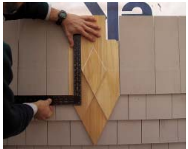
Figure 3. A pair of overlapping point shingles (top) starts the design. The author slips one of these shingles under the housewrap for better water resistance. To build up the diamond pattern, he installs additional point shingles at each course, using a framing square to align them with the point shingles in the previous courses (center, bottom). Note the V-shaped outline drawn on the shingles, which indicates where it is safe to drive fasteners.
