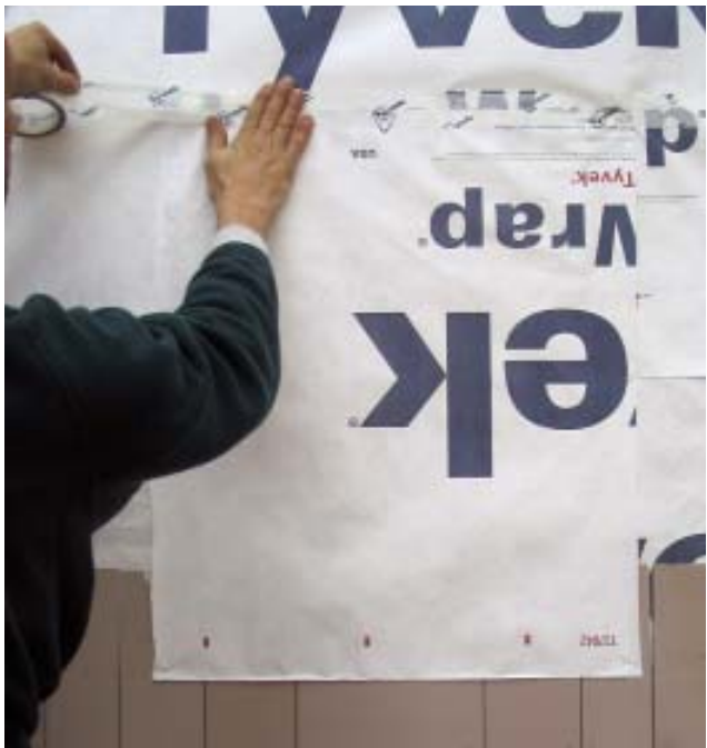
Figure 2. After installing the last full course of straight shingles, the author slits the housewrap above the diamond area. He then slips a piece of the housewrap into the slit (top), which extends about 6 inches beyond the diamond on each side. He tapes the top and trims the bottom so it laps 4 inches over the last full shingle course (bottom).
