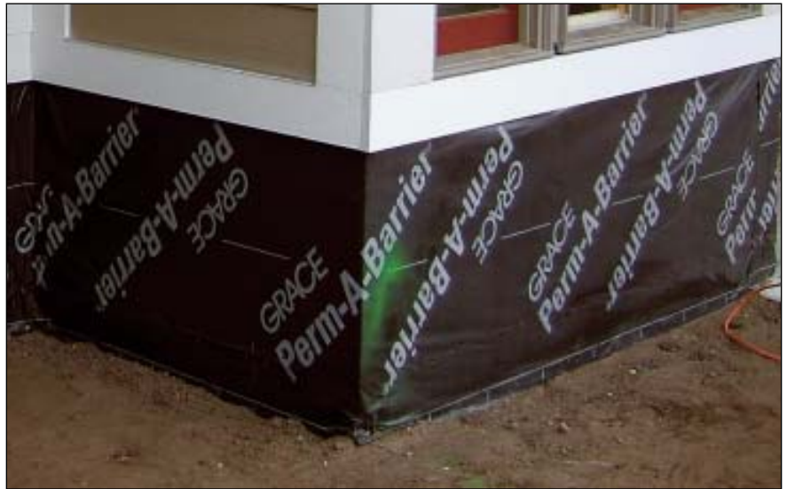
FIGURE 1. The key to wind-smart detailing begins with a continuous air barrier. While ordinary housewrap might work, a self-adhesive membrane applied to continuous sheathing is more durable and less likely to leak once installed. In heating climates especially, it's important to use a specially formulated membrane (or comparable spray-on liquid) that will not create an exterior vapor barrier.
