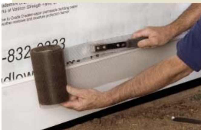
Figure 5. Two 3-inch-wide polypropylene-mesh vent strips — one at the top, one at the bottom — help provide continuous ventilation behind the siding (top and center). For good measure against bugs, the strips were wrapped in insect screening, installed first (above).
