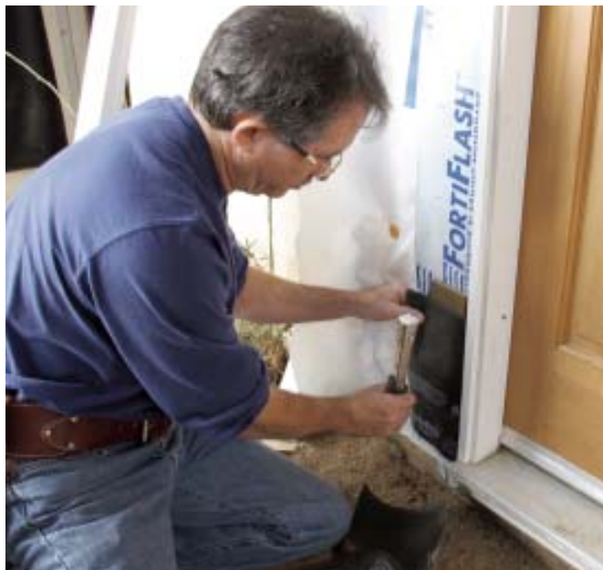
Figure 3. Covering the 1/2-inch plywood spacer with building paper (above) helps prevent water from moving between the wood trim and the plywood block. All cut edges should be primed before installation (left). Note the 1/2-inch jamb extension (below), which brings the back of the trim out flush with the top of the spacer blocks.
