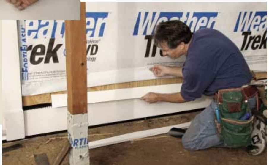
Figure 4. Custom-bent vinyl flashings tuck in beneath the housewrap above doors and windows (top) and at the water table (above and right), bringing any water that reaches the drainage plane back out to the surface.
