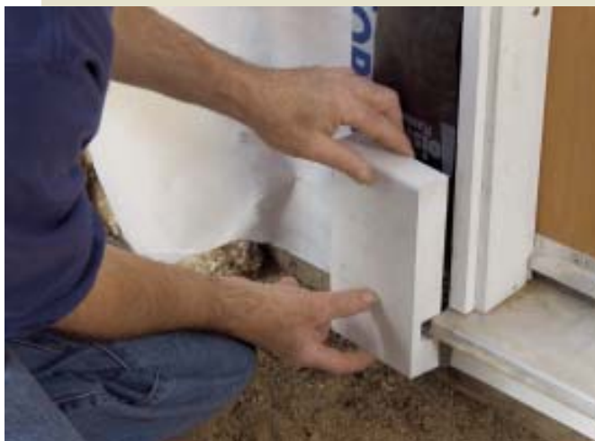
Figure 3. Covering the 1/2-inch plywood spacer with building paper (above) helps prevent water from moving between the wood trim and the plywood block. All cut edges should be primed before installation (left). Note the 1/2-inch jamb extension (below), which brings the back of the trim out flush with the top of the spacer blocks.
