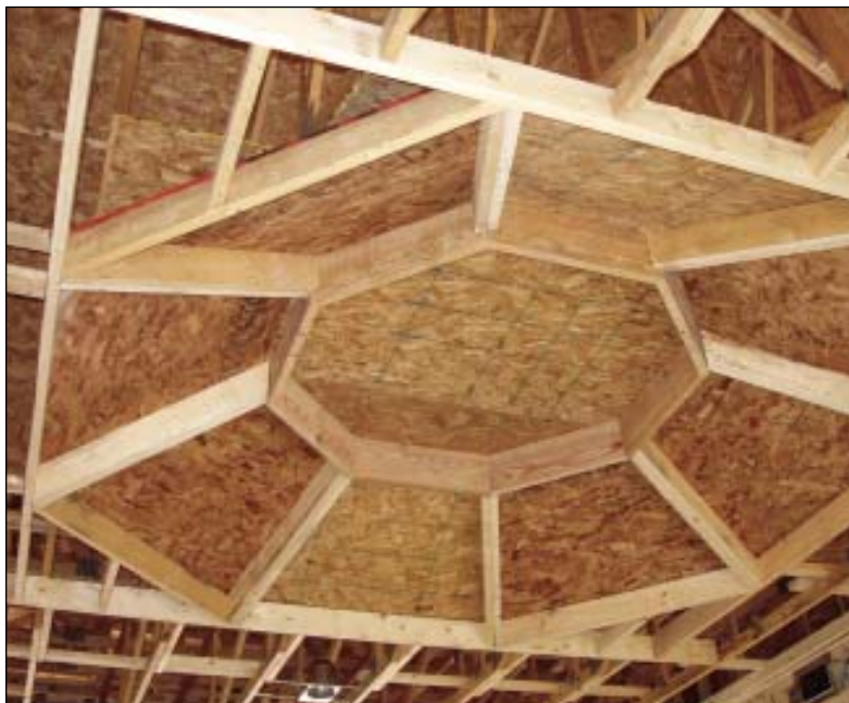
FIGURE 3. Two architectural ceilings framed beneath a truss roof have been backed with OSB. In each case, the OSB isolates the occupied space from the unconditioned attic, providing the insulation subcontractor with simple flat planes on which to apply his attic insulation, instead of forcing him to puzzle out how to fit insulation into complex cavities.
