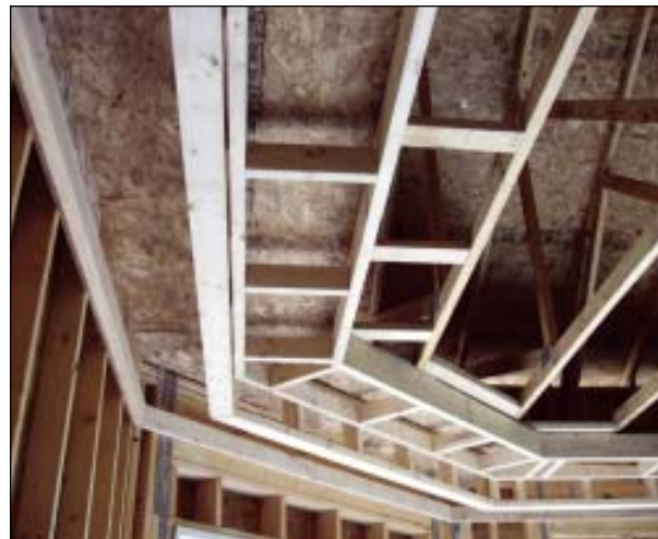
FIGURE 3. Two architectural ceilings framed beneath a truss roof have been backed with OSB. In each case, the OSB isolates the occupied space from the unconditioned attic, providing the insulation subcontractor with simple flat planes on which to apply his attic insulation, instead of forcing him to puzzle out how to fit insulation into complex cavities.
