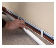
baseboard. When it's time to add wires or move electronic equipment, the homeowners simply pull off the baseboard. Similar products are available for crown molding. WireTracks come in 8- and 5-foot sections, for \$20 and \$14, respectively.
