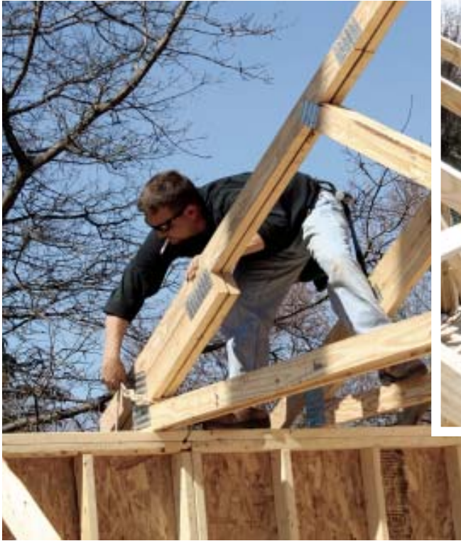
Figure 7. Lifting trusses in pairs eliminates waiting: There's just enough time to set the two trusses, using precut braces marked with the layout (right), while the crane operator picks up the next pair. Unlike longer braces, the 49½-inch-long pieces don't get in the way of the next trusses to be set.
