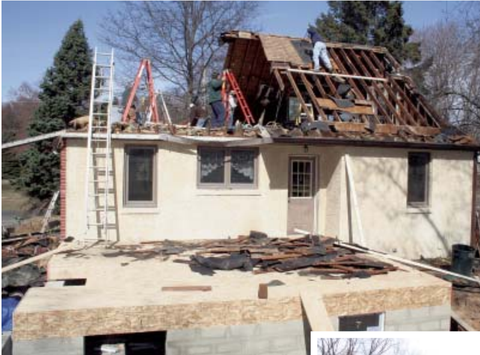
Figure 2. Demo of the existing roof took half a day. A dump trailer provided by the excavation contractor handled the debris.
