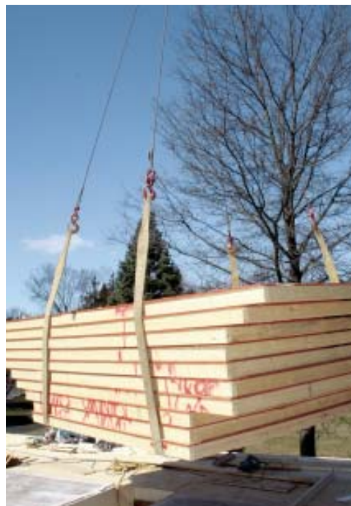
Figure 4. On its first visit, the crane lifted the second-story wall panels onto the deck. Wall framing took a day.
