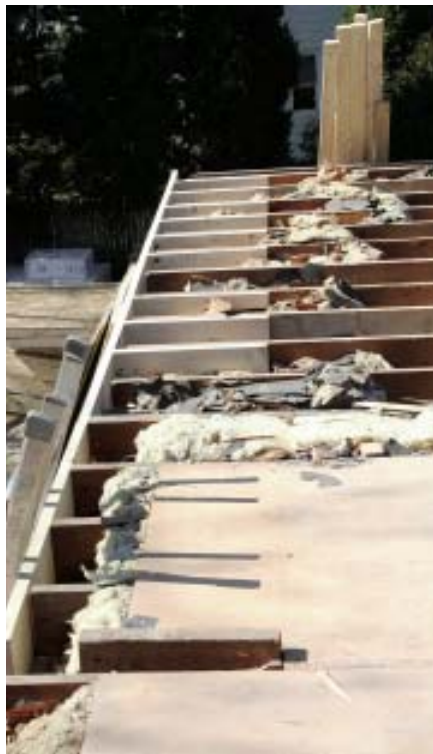
Figure 3. Flooring behind the original upstairs knee walls had to be filled in before the wall panels could be set. Two-by-ten blocks extended the tapered joist ends.
