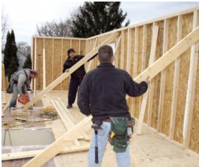
Figure 4. On its first visit, the crane lifted the second-story wall panels onto the deck. Wall framing took a day.
