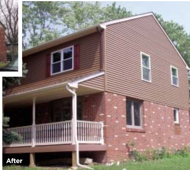
Figure 8. The completed home (left) looks vastly different from the original structure and has 1,000 square feet of additional living space. The family-room addition on the back of the house (below) contains a cathedral ceiling and a wood-burning fireplace.
