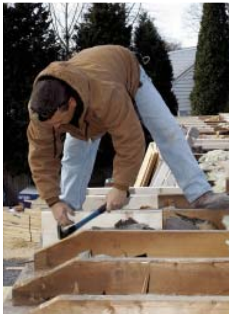
Figure 3. Flooring behind the original upstairs knee walls had to be filled in before the wall panels could be set. Two-by-ten blocks extended the tapered joist ends.
