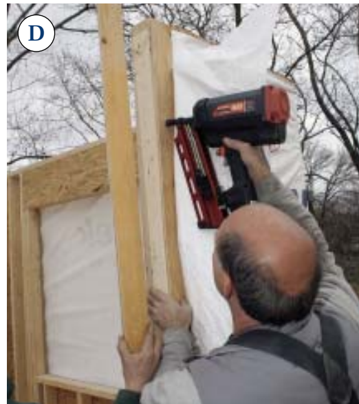
Figure 5. Because the existing floor was 2 inches out of square, the crew had to lengthen one wall panel by removing the last stud (A), cutting off the plate (B), and replacing the stud (C). Another panel was lengthened with plywood spacers (D).
