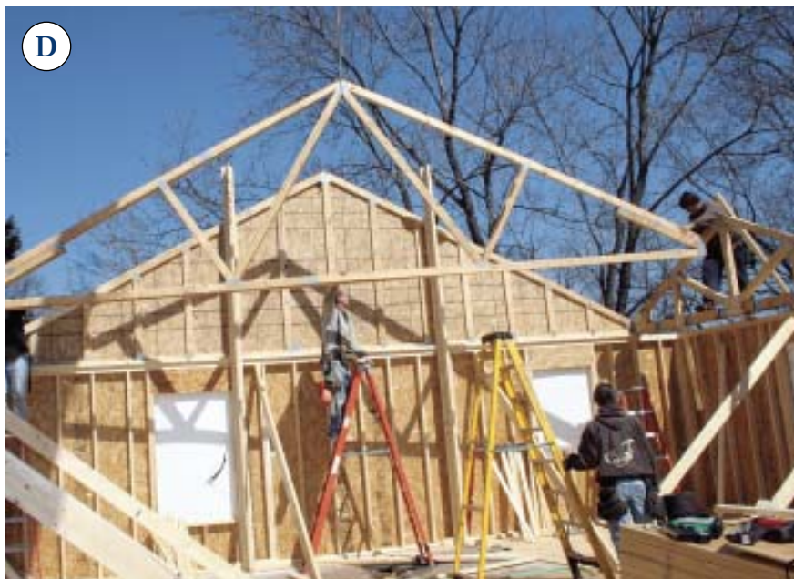
Figure 6. In preparation for the crane's second visit, the crew installed the girder truss for a small bump-out (A). The gable truss was prepped with building paper (B) and pre-installed blocking for the drywall ceiling (C). When the crane arrived, truss-setting moved quickly (D); note the vertical bracing for the gable truss, installed on the inside rather than the outside of the end wall.
