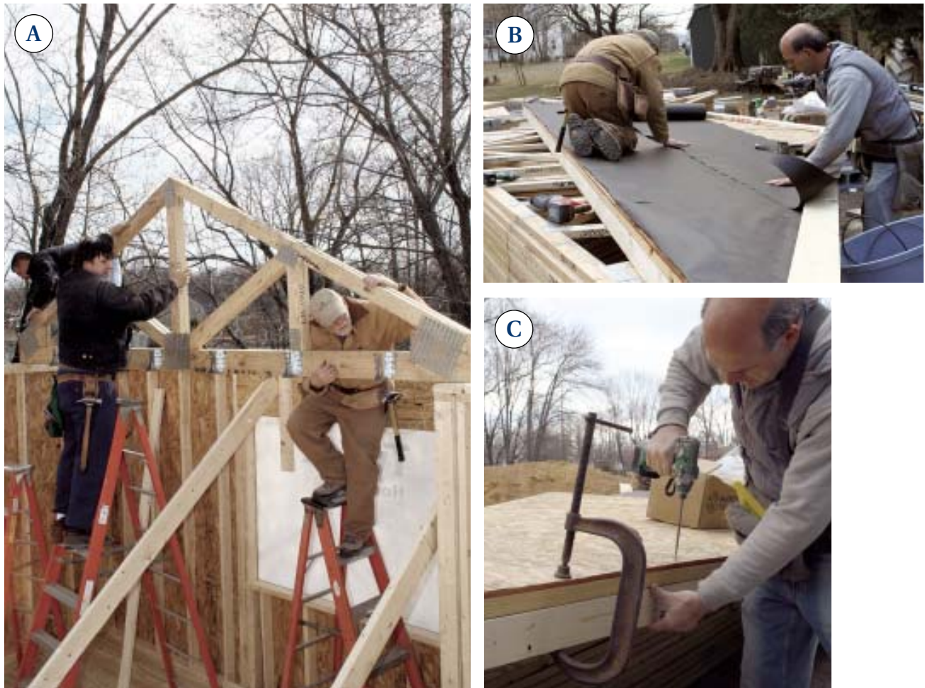
Figure 6. In preparation for the crane's second visit, the crew installed the girder truss for a small bump-out (A). The gable truss was prepped with building paper (B) and pre-installed blocking for the drywall ceiling (C). When the crane arrived, truss-setting moved quickly (D); note the vertical bracing for the gable truss, installed on the inside rather than the outside of the end wall.
