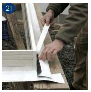
install the head flange before the jamb flanges to avoid creating a reverse lap when the door is upright. I fold one-third of the flange back on itself, remove the release paper from the middle third of the flange, position the piece at the door head, and press it onto the back of the head casing (15). Then I remove the release paper from the folded-back portion of the flange (16), fold this outer third up against the doorframe head, and stick it in place (17).
