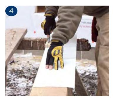
point and work my way uphill, making sure each layer overlaps the previous one and avoiding any reverse laps. In the case of an entrance door, this means I start with the sill flashing.
