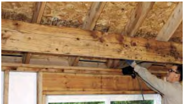
Figure 7. The author's crew frames the opening by carefully trimming the joists in a straight line (above), then nailing on a 2x12 rim board (above right). Rafters will be installed above the line on the rim. On the outside wall, the rim is positioned plumb against the rafters using short nailing blocks (right).
