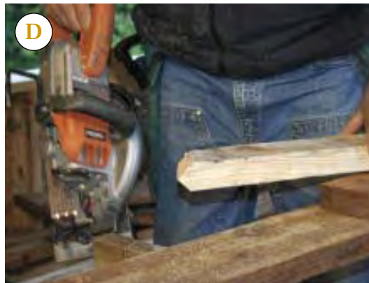
Figure 5. Here, a carpenter lays out the first set of bevel cuts on a hip by drawing parallel lines at the angle of the plumb cut on the hip. The distance between the lines is equal to the thickness of the stock — in this case, 1\frac{1}{2} inches (A). It takes two 45-degree bevel cuts to cut the end of the hip. The first cut is made on the outer line with the blade angled toward the other end of the stock (B). The second cut is on the inner line with the blade angled toward the cut end (C). The result is a 90-degree point (D) in plan view that will fit the inside corner of the opening or between the king commons where they meet at the upper rim.
