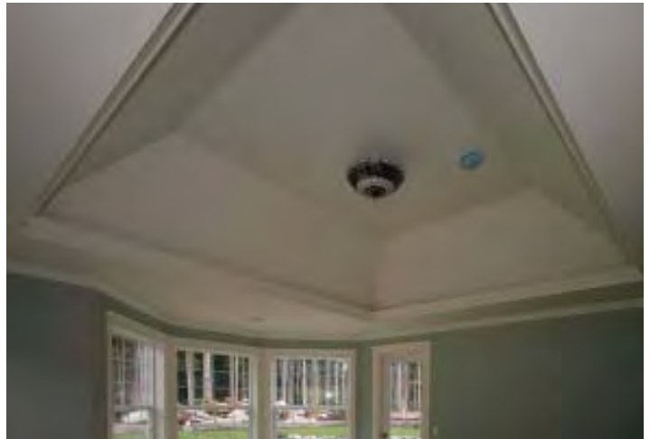
Figure 1. A hipped tray ceiling (above) adds visual interest without a lot of additional framing cost. It's framed like a hip roof except that it's flat on top (right).
