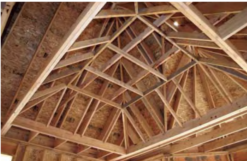
Figure 1. A hipped tray ceiling (above) adds visual interest without a lot of additional framing cost. It's framed like a hip roof except that it's flat on top (right).
