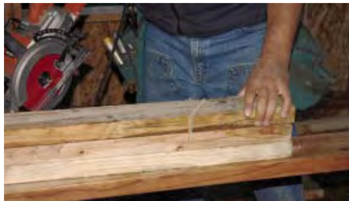
Figure 4. To save time cutting the commons, the carpenters stack the material and score the cut on the second piece while cutting the top piece.
