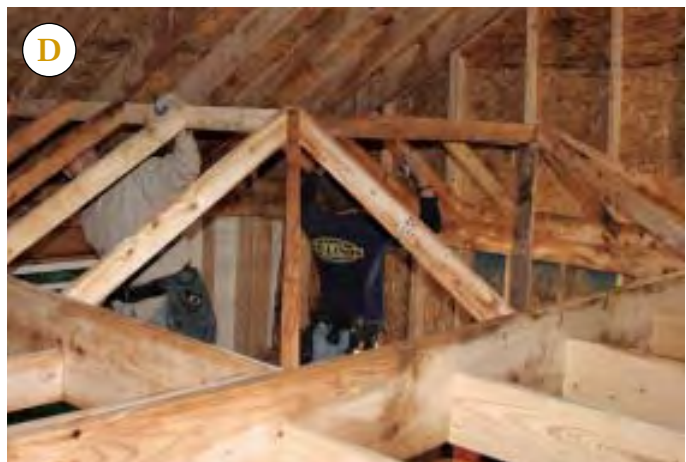
Figure 9. While it's possible to calculate the lengths of the upper rim pieces, the author finds it quicker and easier to install the hips and king commons (A), measure between them (B), and then cut the rim pieces to fit (C). Once the upper rims are in place (D), it's a simple matter to install the commons and run ceiling joists across the top.
