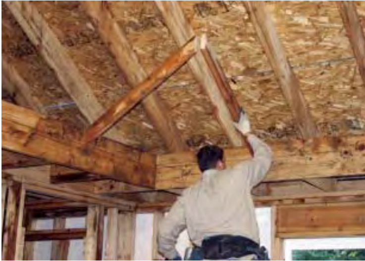
Figure 8. King commons, which flank the hips, are positioned the same distance out from the corner as the run of a common — in this project, 2 feet 5\frac{15}{16} inches (above). The rafters install fast because toenailing holds them in place until the upper rim is installed. After the hips are nailed up (above right), the king commons and hips get nailed together at the top (right).
