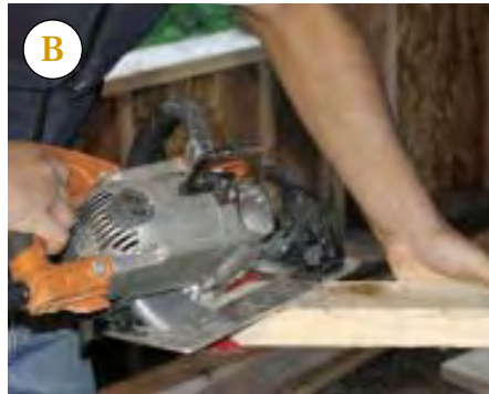
Figure 5. Here, a carpenter lays out the first set of bevel cuts on a hip by drawing parallel lines at the angle of the plumb cut on the hip. The distance between the lines is equal to the thickness of the stock — in this case, 1\frac{1}{2} inches (A). It takes two 45-degree bevel cuts to cut the end of the hip. The first cut is made on the outer line with the blade angled toward the other end of the stock (B). The second cut is on the inner line with the blade angled toward the cut end (C). The result is a 90-degree point (D) in plan view that will fit the inside corner of the opening or between the king commons where they meet at the upper rim.
