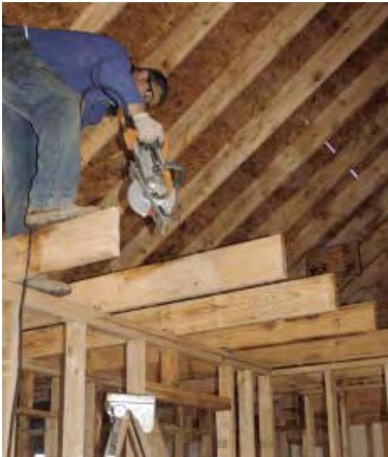
Figure 7. The author's crew frames the opening by carefully trimming the joists in a straight line (above), then nailing on a 2x12 rim board (above right). Rafters will be installed above the line on the rim. On the outside wall, the rim is positioned plumb against the rafters using short nailing blocks (right).
