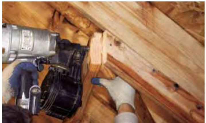
Figure 8. King commons, which flank the hips, are positioned the same distance out from the corner as the run of a common — in this project, 2 feet 5\frac{15}{16} inches (above). The rafters install fast because toenailing holds them in place until the upper rim is installed. After the hips are nailed up (above right), the king commons and hips get nailed together at the top (right).
