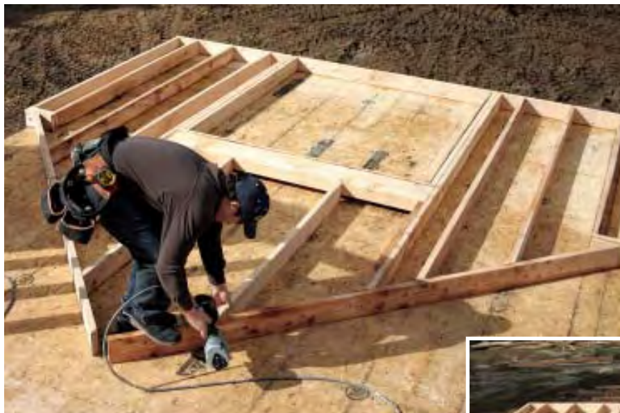
Figure 4. The layout is used to position studs as the wall is assembled. After nailing the studs between the plates (above), the carpenters nail the rake rafters on top of the wall (right). Door and window headers are installed as needed.
