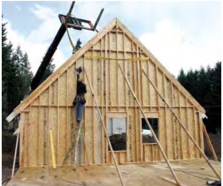
Figure 8. To prepare this wall for lifting, the author's crew puts a heavy lifting strap through holes in the sheathing, runs it across the inside face of the studs, then loops the ends onto the forks of an all-terrain forklift (top left). A carpenter uses hand signals to direct the forklift driver as he lifts the wall (top right). The crew quickly plumbs and braces the wall with prepositioned diagonal braces (above).
