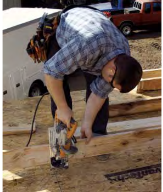
Figure 3. The full-size layout is used to mark the bevel cuts on rake studs. These studs have been placed on the stud layout; they butt to the bottom plate so the carpenter can mark where they cross the line representing the underside of the top plate (above). With the saw set to the bevel angle of the roof, the author cuts rake studs to length (right).
