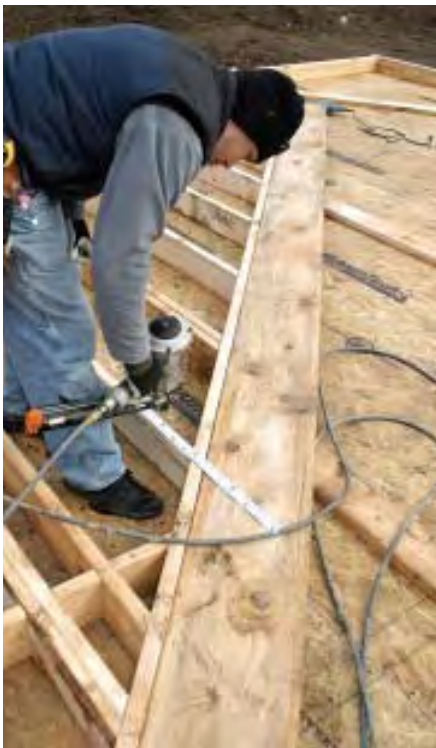
Figure 6. Metal straps (top) function as hinges to prevent the wall from sliding off the deck during lifting. On large walls, the crew installs reinforcing straps (above left) next to the studs where the lifting straps will go. Carpenters sheathe the wall in the usual way, then use a powerful router with a flush trimming bit to cut out openings (above right).
