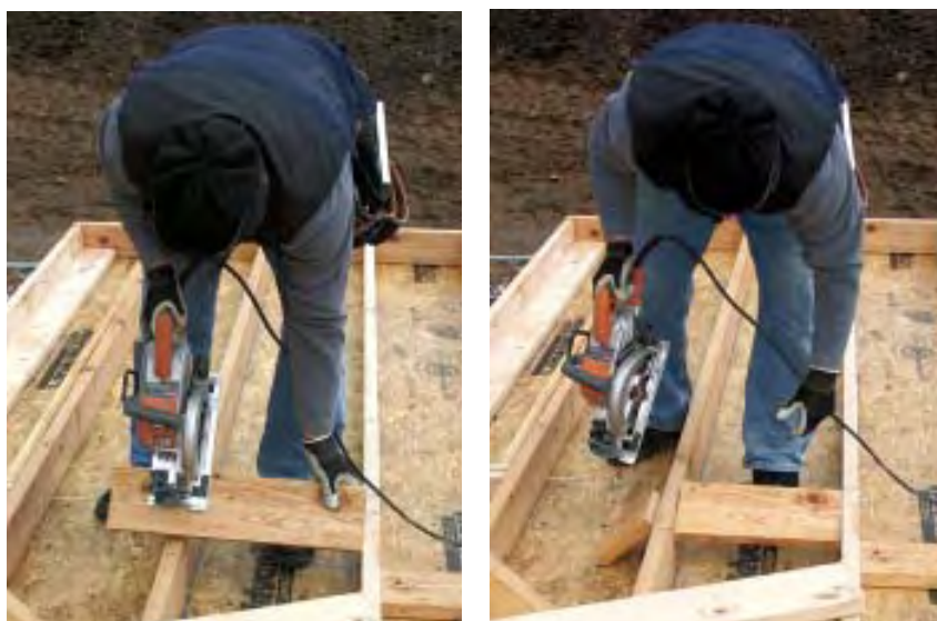
Figure 5. Rather than waste time measuring blocking with a tape, a carpenter lines up the saw by eye and makes the cut.
