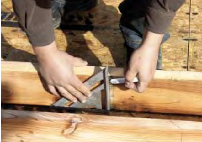
Figure 3. The full-size layout is used to mark the bevel cuts on rake studs. These studs have been placed on the stud layout; they butt to the bottom plate so the carpenter can mark where they cross the line representing the underside of the top plate (above). With the saw set to the bevel angle of the roof, the author cuts rake studs to length (right).
