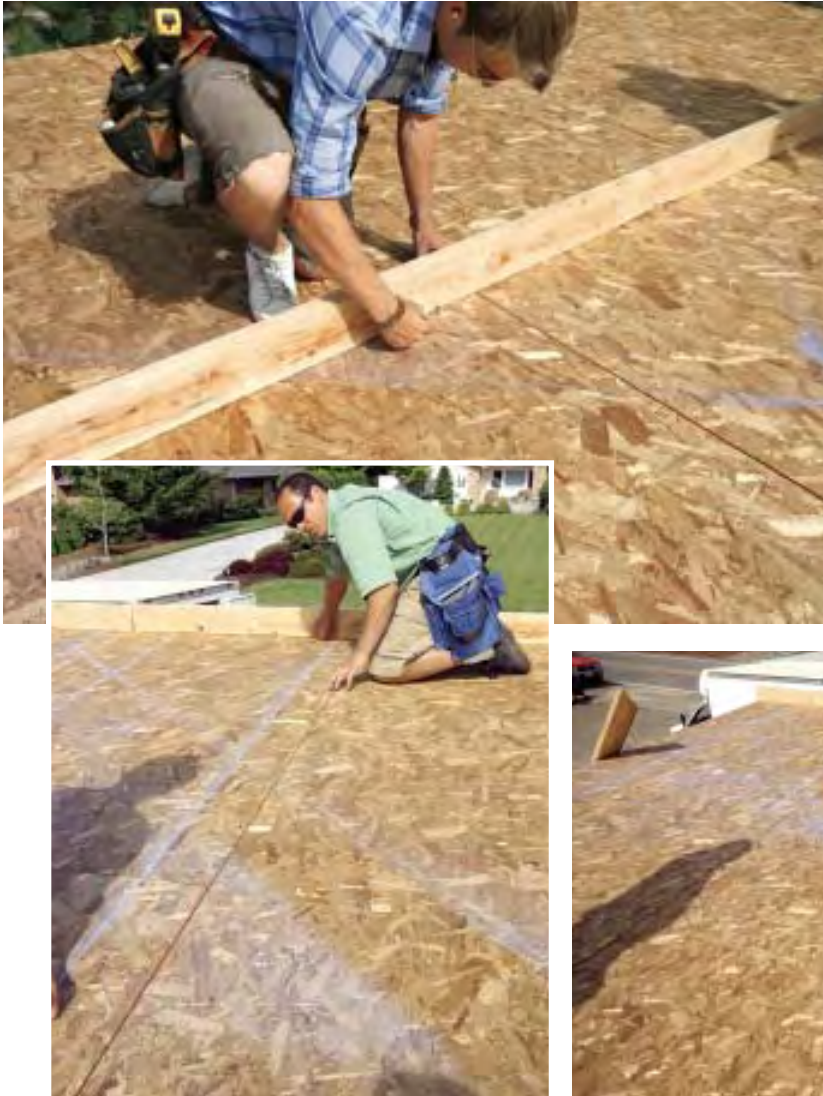
Figure 1. The bottom plate does double duty as a story pole for transferring the rake-wall stud layout farther up the deck (left). After tacking the plate to the deck, the crew snaps lines between the layout marks (below left) to indicate where each stud will go. The finished layout (below) is a full-size template for marking cuts and assembling pieces. There's no stud marked in the middle of this wall because there will be an opening there.
