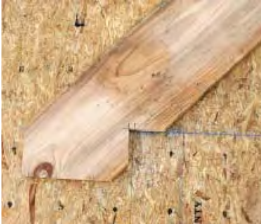
Figure 2. The author cuts a pair of rafters and tacks them down over layout lines or against the actual corner pieces of the wall. On this layout (above), the blue line represents the top of the wall and the pencil line represents the face of a stud. With the rafters in position (above right), the author scribes a line along the bottom to mark the upper edge of the top plate. To mark the lower edge, he removes the rafters and snaps a parallel line 1½ inches in from the scribed one (right).
