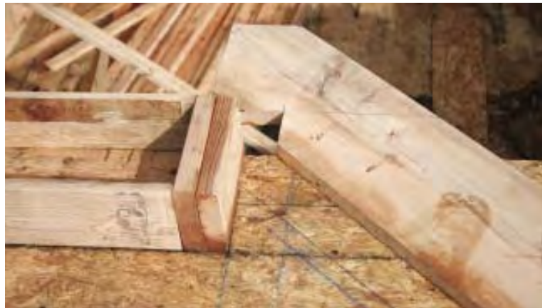
Figure 2. The author cuts a pair of rafters and tacks them down over layout lines or against the actual corner pieces of the wall. On this layout (above), the blue line represents the top of the wall and the pencil line represents the face of a stud. With the rafters in position (above right), the author scribes a line along the bottom to mark the upper edge of the top plate. To mark the lower edge, he removes the rafters and snaps a parallel line 1½ inches in from the scribed one (right).
