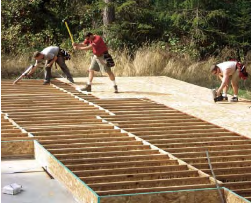
Figure 9. When installing the sub-floor, everyone has a particular job: One carpenter does nothing but glue, two carpenters cut and place the sheets and beat them together, and one just nails.
