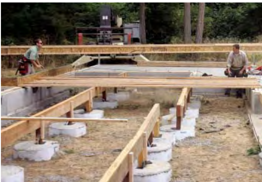
Figure 6. After the girders are in, the crew installs rim boards (top), then places the joists in rough position (above).
