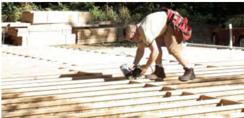
Figure 8. To finish the frame, the author nails joists to the rim (top left) and sill (top right), then installs the required blocking (above).
