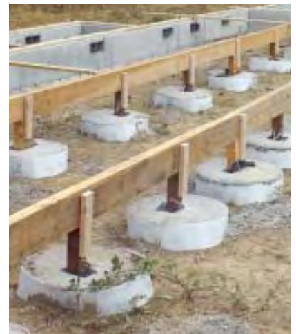
Figure 5. With a crawlspace foundation, the author uses girders to break up the floor span. Instead of measuring, the crew lays the girder stock in rough position (above) and cuts the pieces so the joints land over footing pads (above right). The girders are supported by posts that land on pieces of rubber membrane and are tied to the footings with cast-in straps (right).
