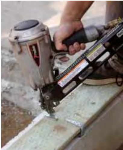
Figure 4. Fastening sills with cast-in strap anchors (above left) is faster than using anchor bolts. The carpenters place the sill stock on layout, tack it in place with a powder-actuated fastener (above), then fasten it by nailing on the strap (left).
