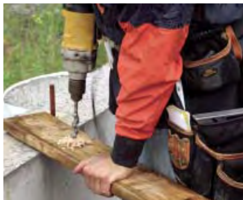
Figure 3. A carpenter butts sill stock to the bolts, squares in from them (right), then measures the distance between each bolt and the layout line (far right, top). After marking that distance on the stock, he drills the bolt holes (far right, bottom).
