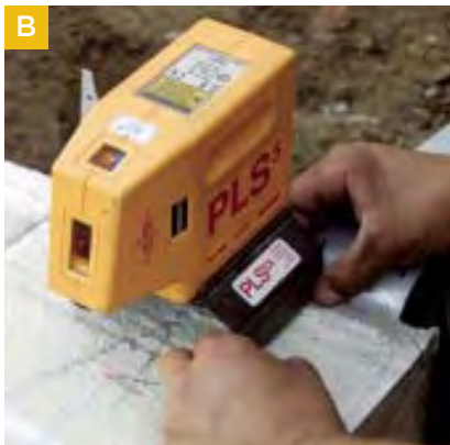
Figure 1. Crew members snap sill layout on the longest wall of the foundation (A), mark the inside corner, and align the laser over that point (B). Next, they place a target over the line at the far end of the wall and rotate the laser until the front beam hits the target dead center (C). Finally, they locate the perpendicular line by placing the target on the adjoining wall so that the side beam hits it dead center (D), mark that location, and measure in one inch to account for the offset between the down beam and side beam on the PLS5 laser. A line between this point to the inside corner will be square to the original line (E).
