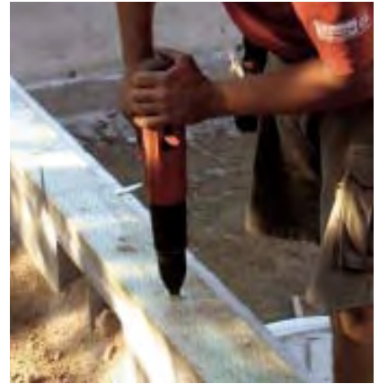
Figure 4. Fastening sills with cast-in strap anchors (above left) is faster than using anchor bolts. The carpenters place the sill stock on layout, tack it in place with a powder-actuated fastener (above), then fasten it by nailing on the strap (left).
