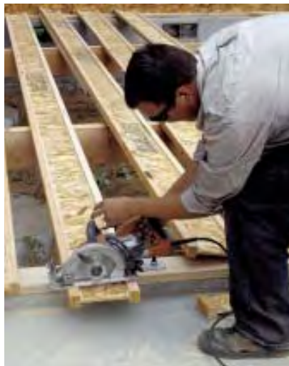
Figure 7. Rather than measuring each joist, a carpenter butts them all to the opposite rim, snaps a line where the inner face of the rim will be (far left), and then cuts them in place with a circular saw (left).
