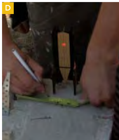
Figure 1. Crew members snap sill layout on the longest wall of the foundation (A), mark the inside corner, and align the laser over that point (B). Next, they place a target over the line at the far end of the wall and rotate the laser until the front beam hits the target dead center (C). Finally, they locate the perpendicular line by placing the target on the adjoining wall so that the side beam hits it dead center (D), mark that location, and measure in one inch to account for the offset between the down beam and side beam on the PLS5 laser. A line between this point to the inside corner will be square to the original line (E).
