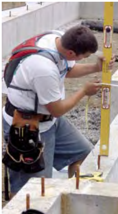
Figure 2. To lay out sills on a stepped foundation, most carpenters stretch the tape horizontally and use a level to plumb down (left). A faster method is to stretch the tape, position the laser so the up beam hits the desired mark (above), then mark where the down beam hits the foundation.
