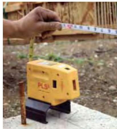
Figure 2. To lay out sills on a stepped foundation, most carpenters stretch the tape horizontally and use a level to plumb down (left). A faster method is to stretch the tape, position the laser so the up beam hits the desired mark (above), then mark where the down beam hits the foundation.
