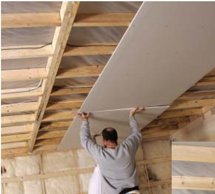
Figure 7. The author prefers to install drywall perpendicular to the framing. Not only does this give the structure greater strength, but the drywall can float over slightly uneven joists and studs, making them less conspicuous. In the photo at right, the second course of drywall bridges the flush beam, which will have no screws installed in it.
