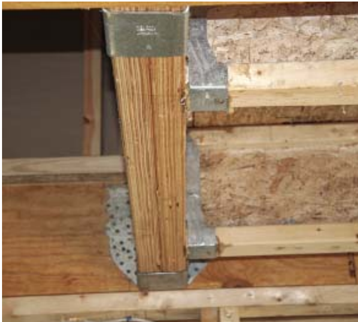
Figure 5. Low joist hangers can create problems for the drywall. Notching the ends of the joists, as was done here, gets them up out of the way.
