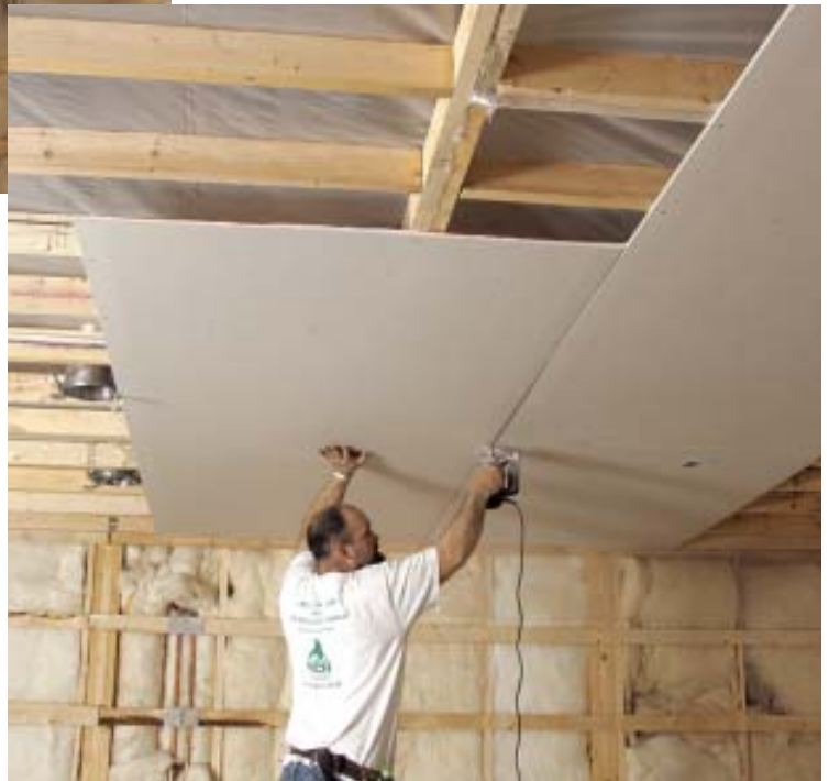
Figure 7. The author prefers to install drywall perpendicular to the framing. Not only does this give the structure greater strength, but the drywall can float over slightly uneven joists and studs, making them less conspicuous. In the photo at right, the second course of drywall bridges the flush beam, which will have no screws installed in it.
