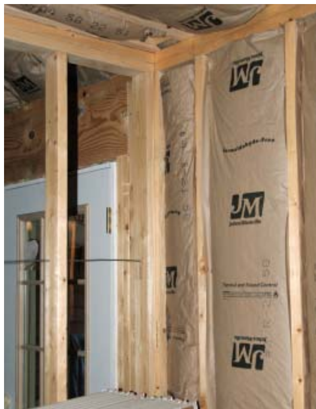
Figure 6. Sagging and overstuffed insulation (top) can make it difficult to get drywall snug to the framing, leading to ridged seams and popped screws. Face-stapling wall batts also makes it hard to fasten drywall tightly. Inset-stapling, as shown (above), solves the problem but is not liked by energy-efficient builders. An alternative is to use unfaced batts and a poly vapor retarder.
