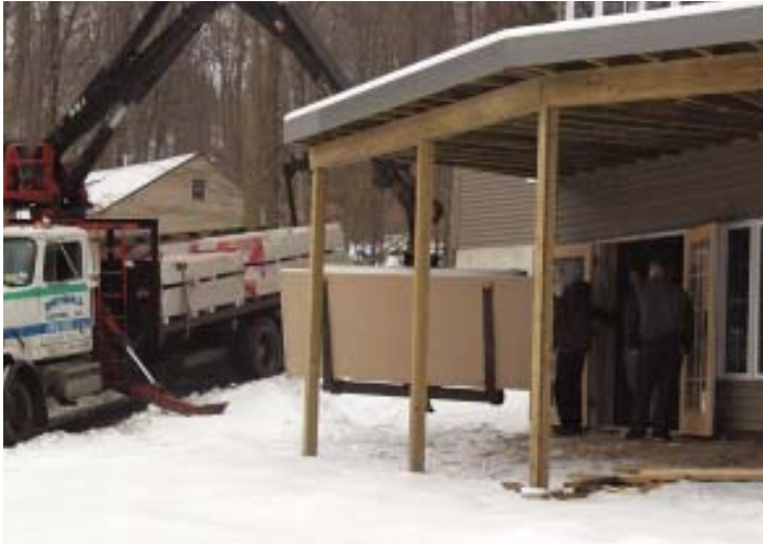
Figure 1. A boom-truck delivery saves a lot of carrying, so make sure that site conditions allow the truck to get next to the house.
