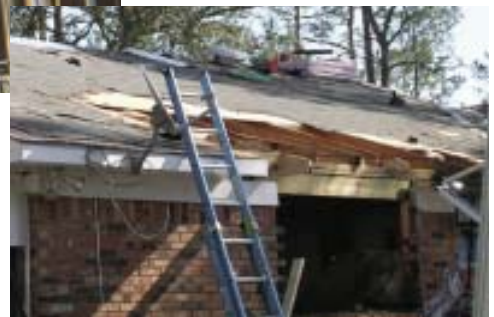
Students from Birmingham-Southern College tear off a house's old asphalt roofing (above). Before the new roof could be put on, hurricane-damaged rafters and sheathing had to be replaced (right).
