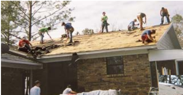
Students from Birmingham-Southern College tear off a house's old asphalt roofing (above). Before the new roof could be put on, hurricane-damaged rafters and sheathing had to be replaced (right).
