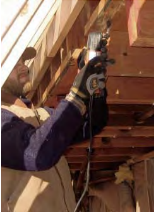
Figure 4. After determining that the 8½-inch-deep beam wouldn't fit within the home's existing floor system, the author used a Fein MultiMaster to remove the subfloor for an additional ⅝ inch of clearance (above). Here, the opening is ready to receive the beam (above right).
