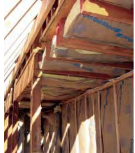
Figure 2. A 2x10 ledger fastened to the studs with 1/2-inch lag screws serves as an attachment point for the 2x8 diagonal braces (above left). A second ledger beneath the top end of the braces keeps them snugly in place and helps prevent splitting. A sheathed, insulated 2x4 wall on the inside picks up the second-story floor loads (above).
