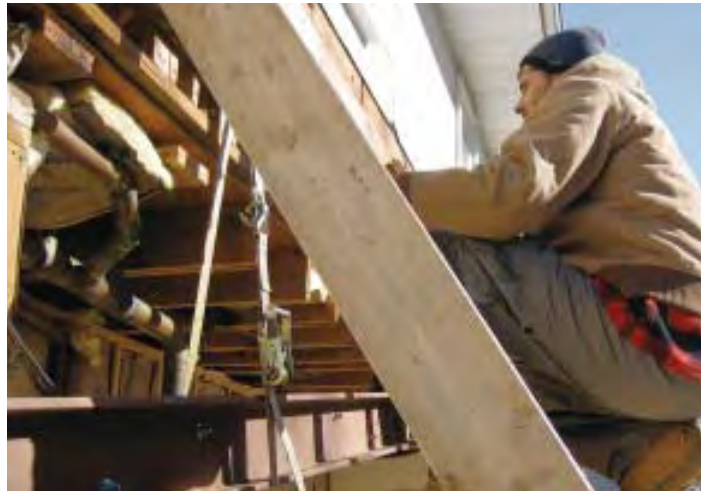
Figure 5. A chain hoist attached to the temporary ledger supplied lift (top photos). After the hoist maxed out, a pair of heavy-duty ratchet straps finished the job (above).
