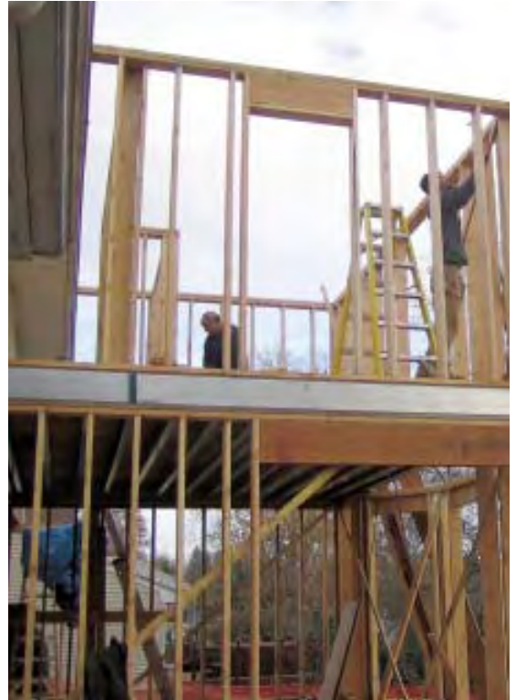
Figure 8. Eight-inch-deep steel joists on 12-inch centers provide a clear-span ceiling in the kitchen. The doubled joists on the right side of the photo at left support the whirlpool tub. The steel band joist is visible between floors (above).
