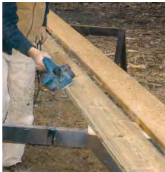
Figure 3. A sandwich of pressure-treated lumber and plywood bolted to one side of the I-beam provides a nailer for joist hangers (far left). Knocking the corners off the 2x8 allows it to sit tight to the I-beam's web (left).
