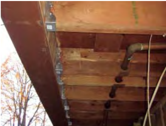
Figure 7. The author used conventional face-mount hangers nailed to the header to support the joist ends on the existing part of the house (above). With the hangers installed and the post bases fastened to the foundation, the ledger and 2x8 supports came down. The temporary wall was left in place to keep the house clean and offer weather protection (right).
