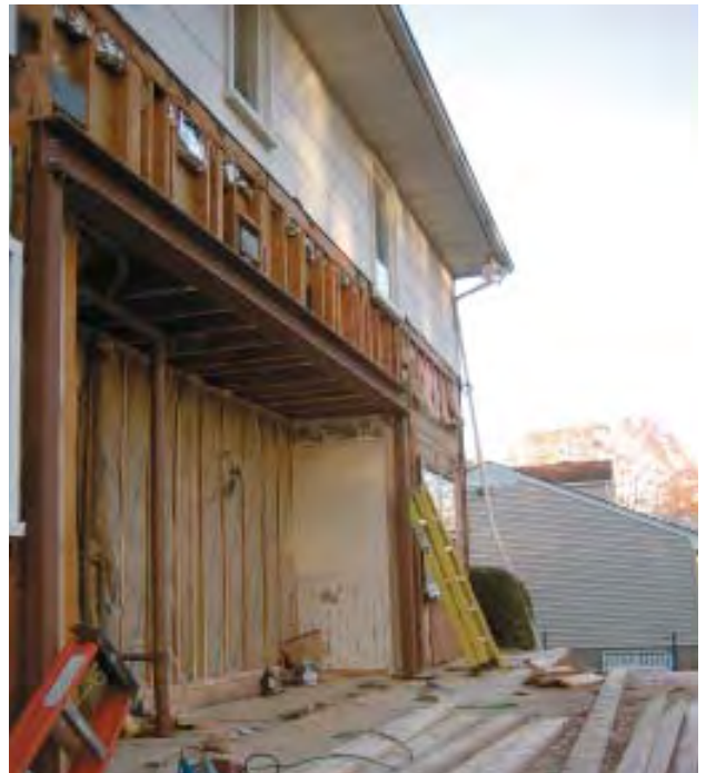
Figure 7. The author used conventional face-mount hangers nailed to the header to support the joist ends on the existing part of the house (above). With the hangers installed and the post bases fastened to the foundation, the ledger and 2x8 supports came down. The temporary wall was left in place to keep the house clean and offer weather protection (right).
