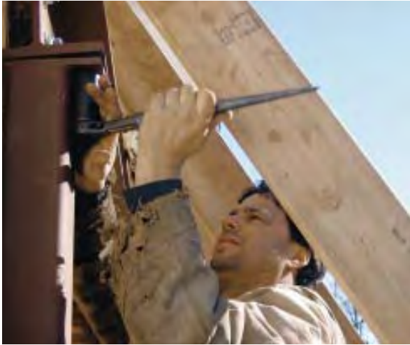
Figure 6. Four-inch steel columns with welded caps and base plates support the beam at each end. Note the 1/2-inch-drive ratchet's drift handle, used for lining up the predrilled bolt holes (above). The column bottoms (above right) would be secured later with one 1/2-inch wedge anchor each; the inside hole landed too close to the edge of the concrete for drilling.
