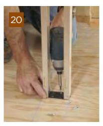
fasten with  $1^{1}/2$ -inch screws (18). Plumb the split-stud pair to the floor (19), then fasten the plate, centered between the snap lines (20). Use Tapcons or anchors on concrete.
