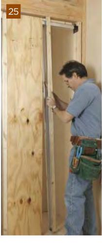
near the top or the bottom of the slot, so as to leave as much room as possible for fastening the split jamb to the split stud later. When using a plywood stiffener, I install the second (midspan) split-stud pair after the plywood is attached to the first split stud (25); I secure the second split stud to the header, then to the plywood, then to the floor.
