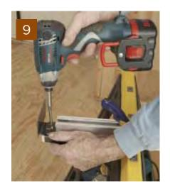
jigsaw to cut the wood (7) and a hacksaw to cut the track (8), then reinstall the end plate (9).
