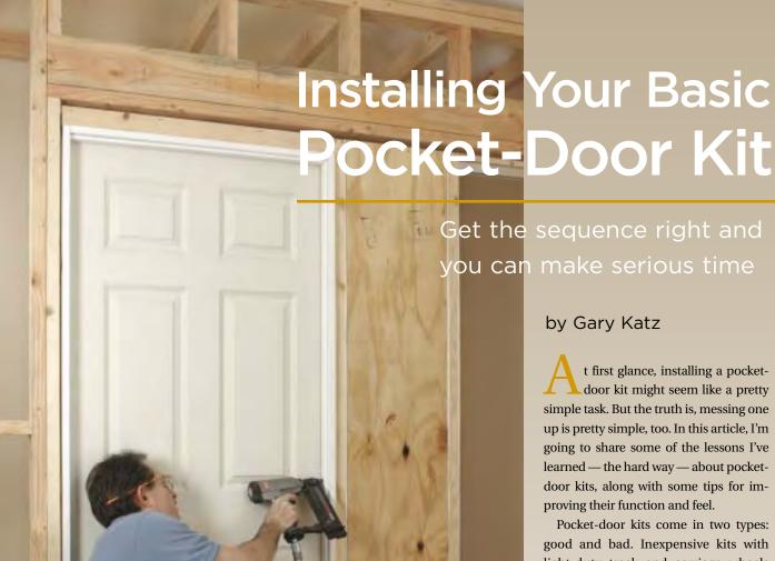
Pocket-door kits come in two types: good and bad. Inexpensive kits with light-duty track and carriage wheels (sometimes called "trucks") are the bane of door-hangers and homeowners. Not only are they difficult to install, but in no time at all the track bends or the wheel bearings wear out. And everyone knows fixing a pocket door isn't easy or cheap.
