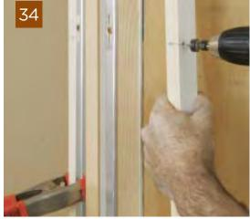
cutouts in the aluminum frames (34). To position the split jambs properly, use a spacer the same thickness as the drywall or other finish wall material (35).
