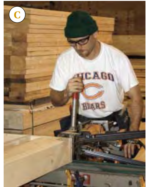
Figure 5. At the framing table, the subcomponents are the first pieces fastened to the plates, along with any cripple studs (A). Steel fingers (painted yellow) ensure accurate 16-inch o.c. spacing and can pivot to lay flat when they interfere with the placement of a double stud, tee, or header (B). Once the remaining studs are placed, the whole panel is held together with pneumatic rams while it's nailed off with special weight-assisted two-gang framing nailers (C). Before the panel moves on, any twisted studs are pried into place with a tweaker (D) before being nailed with a pneumatic nailer; blind cavities are filled with insulation (E).
