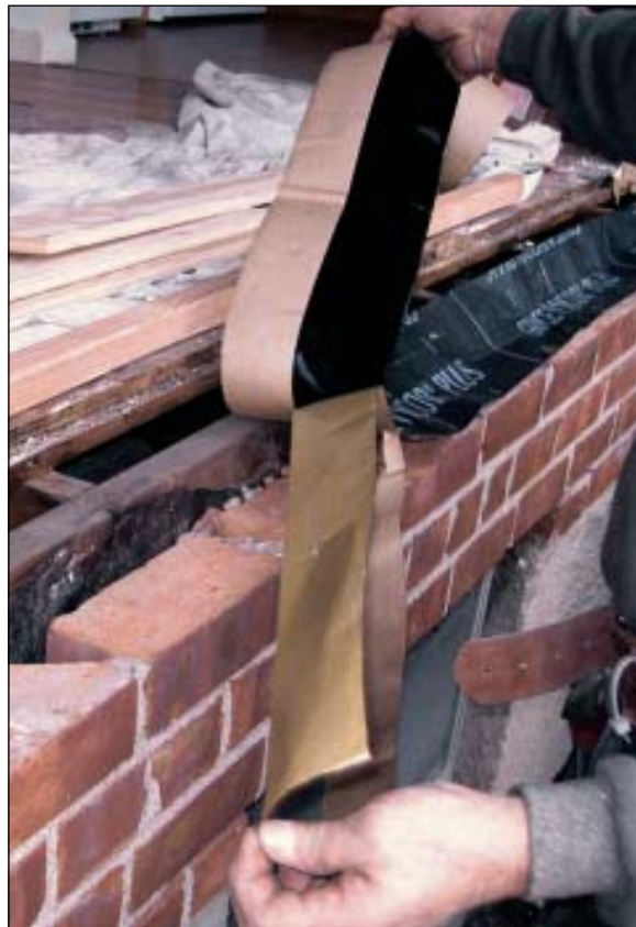
FIGURE 2. Deck-level sliding doors are susceptible to water and air infiltration. To reduce problems, the author begins with a layer of self-adhesive flashing beneath the subfloor and lapped onto the brick veneer.
