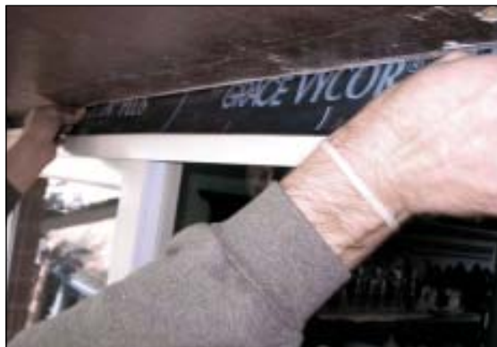
FIGURE 5. Even though a deep overhang protects the head jamb of this opening, the author takes care to seal the head as well (above). He's learned from experience that unless this is done, someone will inevitably power-wash the exterior and inadvertently create a leak.
