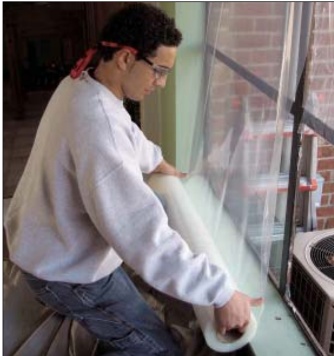
FIGURE 1. Carpet Protection — a strong, self-adhesive plastic film — adheres well to glass (above). When it's applied to both sides of the window, the glass can be broken out without creating a hazard (right).
