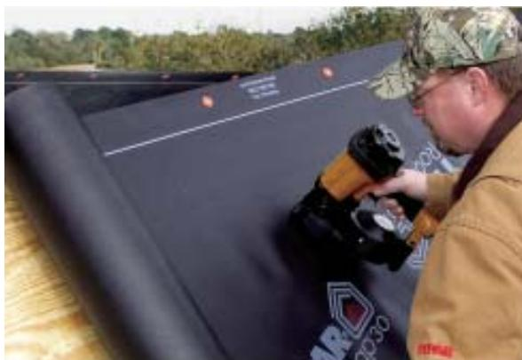
**Do-It-All Wrap.** Typar touts its polypropylene *RoofWrap 30* as an ideal underlayment for shingles, cedar shakes, tile, slate, and metal. Polypropylene underlays tend to have excellent tear resistance and won't crack or become brittle in cold temperatures. The company covers *RoofWrap 30* with a 20-year warranty when it's installed according to the instructions. A 41 $\frac{1}{2}$ -inch 10-square roll weighs about 30 pounds and sells for between \$120 and \$150.
