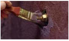
Liquid waterproofing membranes that meet ANSI 118.10 specifications can be applied to the surface of many tile substrates, including cement-based backerboard, plywood, and concrete. Waterproofing membrane should be applied to setting-bed edges, too, and around any plumbing that penetrates the substrate.
