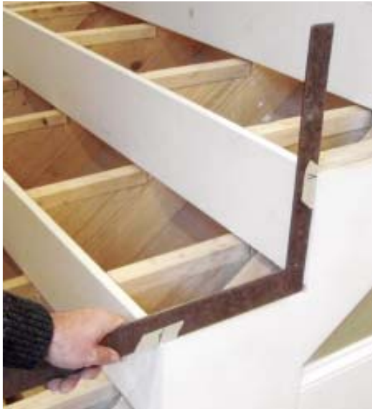
Figure 1. The key to the Up System is an accurate measurement of the stair's rise and run. Here, the author lays a framing square onto a tread and transfers these dimensions to the square (above). Next, he places the framing square on a piece of paper or a scrap of plywood and draws a full-scale right triangle, with the base of the triangle equal to the stair's run and the height of the triangle equal to the stair's rise (right).
