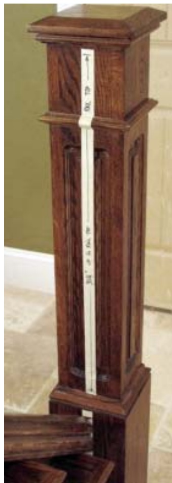
Figure 4. To determine post lengths, the author indicates his preferred handrail location at the top of the post by marking the position on a piece of tape; then he marks the 30 \frac{1}{4} -inch Up number below (left). After laying a section of handrail in position against the post and along the nose of the treads, the author marks the top of the post; this difference is the amount the post needs to be shortened (drawing, above).
