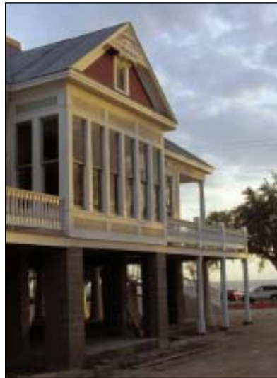
FIGURE 5. Justine now sits on steel piles. The majority of the pilings were encased by concrete masonry units to FEMA specification (left and below), then stuccoed. In front, behind the stairs, tapered columns were constructed of brick and then stuccoed using a 2x4 as a screed and an adjustable metal ring as a template. The finished columns can be seen in the lead photo (page 2).
