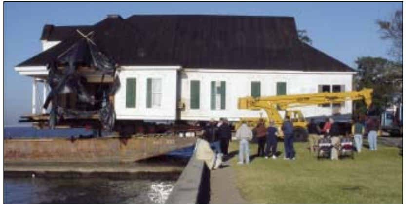
FIGURE 4. On its way to Lake Pontchartrain and eventually to its resting place on Lakeshore Drive in Mandeville, Justine, supported on a grid of steel, is pulled upriver on a barge (above). At the Mandeville seawall (right), the entire home is rolled off the barge and towed across the street to the corner of Gerard Street and Lakeshore Drive.
