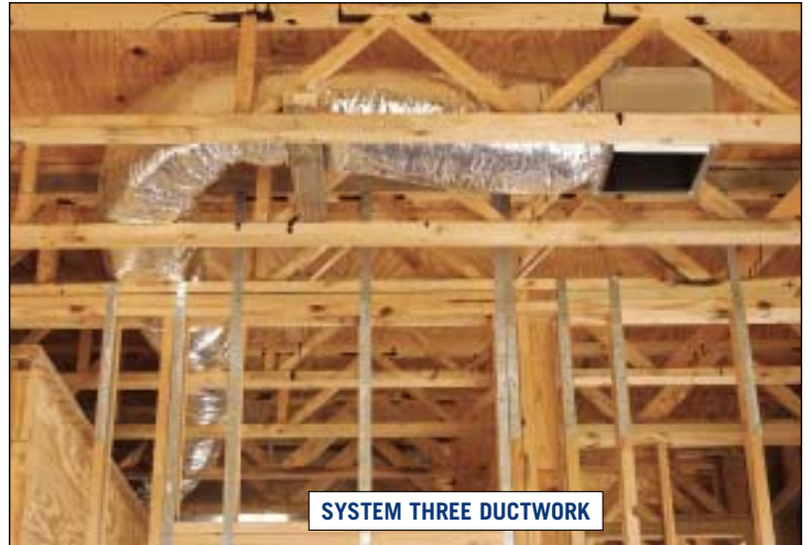
FIGURE 4. In a hot, humid climate, heat and moisture picked up by poorly insulated, leaky ductwork in attic spaces can boost a home's annual cooling loads by 30% or more. The solution is to run ducts through conditioned spaces, such as an insulated attic (left) or through open-web floor trusses (below).
