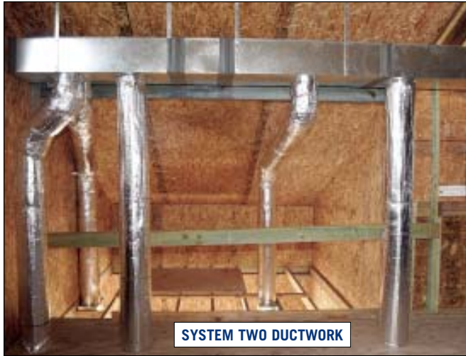
FIGURE 4. In a hot, humid climate, heat and moisture picked up by poorly insulated, leaky ductwork in attic spaces can boost a home's annual cooling loads by 30% or more. The solution is to run ducts through conditioned spaces, such as an insulated attic (left) or through open-web floor trusses (below).
