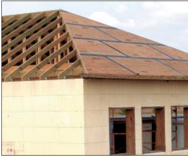
FIGURE 1. The first step in keeping any home cool is providing a thermally efficient building shell. The LaHouse provides several structural systems that optimize insulation, including insulating concrete form walls (above), structural insulated panels (top right), and “advanced framing” — a lumber-conserving, energy-efficient system using 2x6 studs spaced 2 feet on center that were eventually packed with spray cellulose insulation (right).
