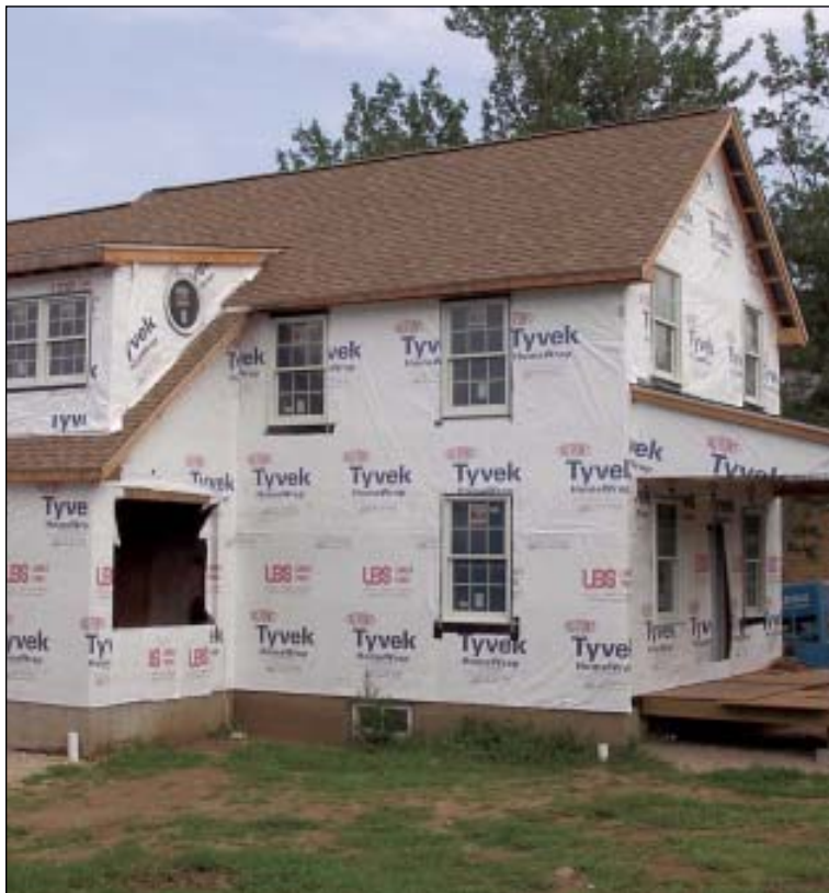
FIGURE 3. Contractor Craig Caulkins of Caulkins Building & Design in Niantic, Conn., routinely applies 1/2-inch or 1-inch Dow Styrofoam to home exteriors under vinyl siding (above right). While foam is water resistant and provides a good barrier against the bulk of the weather, wind-driven rain can find its way around panels and through joints, so Caulkins relies on a housewrap and careful window flashing installed over a fully sheathed structure before installing the foam (above left).
