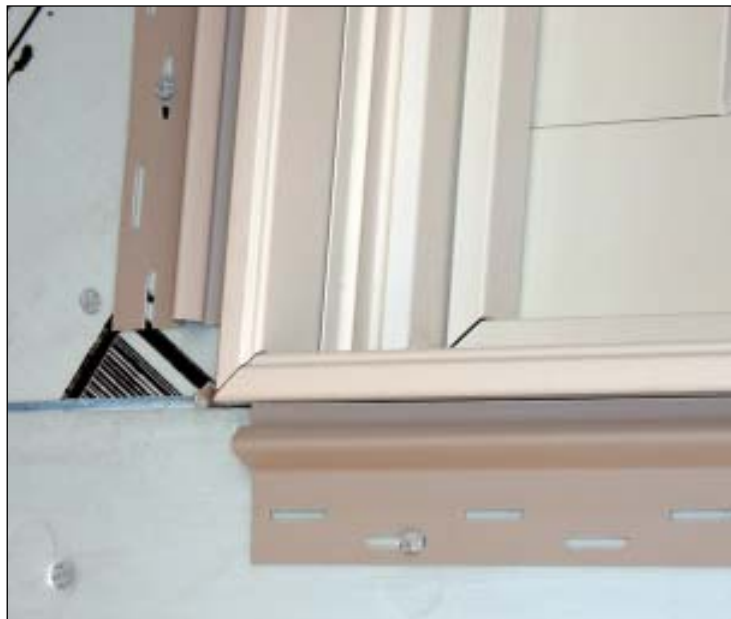
FIGURE 4. In combination with Andersen flanged vinyl windows, says Caulkins, no special furring or attaching method is required: window flanges extend far enough from the wall to cover all foam edges. Crews flash the window openings with self-adhering membrane, fasten the window directly to OSB-sheathed wall, and then apply a two-piece window surround from CertainTeed. The base piece of the window surround is nailed through the foam into the window rough frame (above left), and the matching top piece snaps into place over it (above right).
