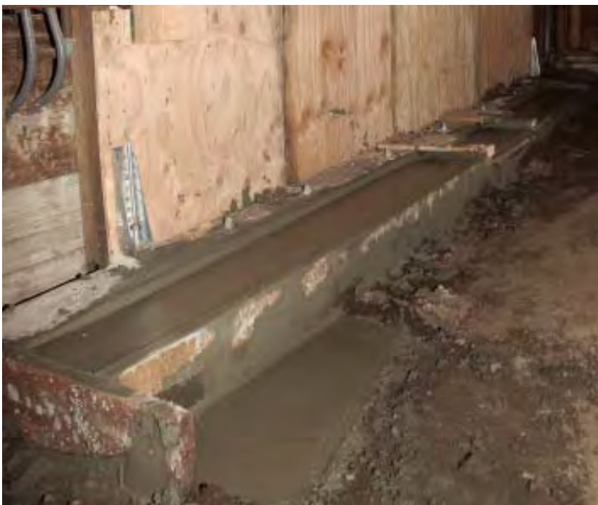
Figure 9. The foundation under this shear wall can support the vertical load but is too weak and shallow to accept hold-downs. Instead of replacing it, the author poured a new reinforced footing alongside the existing one. To tie into the new footing, the hold-downs and anchor bolts are on the interior face of the wall and attached through a “reversed” mudsill. The crew nailed the plywood to the back of the mudsill before standing it up and nailing it to the studs.
