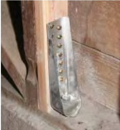
Figure 5. Now that hold-downs are installed, this wall will be sheathed with plywood and turned into a shear wall. The hardware is necessary where a wall is tall enough that overturning forces could result in uplift. It isn't needed on shorter cripple walls.
