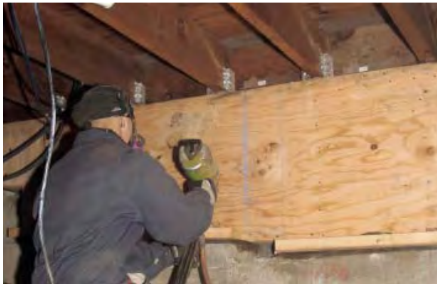
Figure 8. With the anchor bolts and framing hardware installed, this carpenter finishes the job by sheathing the cripple wall with plywood. For best results, use at least 15/32 Structural 1-grade 5-ply plywood.
