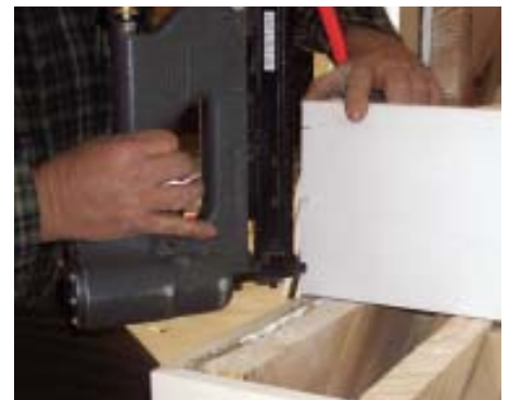
Using Senclamps to fasten long miters is faster than cross-nailing and holds better.
