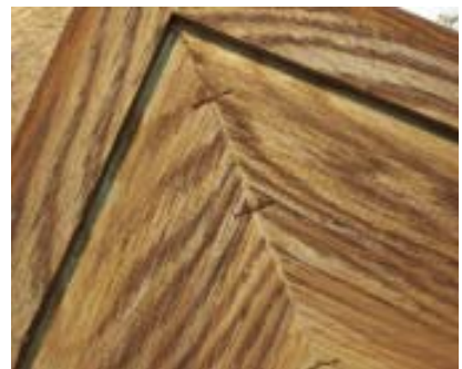
Flat casings are preassembled face-down on the bench. The fasteners aren't visible on the final installation because the author drives them across the back of the joint.
