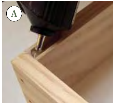
Figure 7. A spot of hot-melt adhesive (A) at either end of the parting bead groove provides fast installation of the bead, which — like the sill — has horns. A wood stop-gauge sets an accurate casing overhang for the parting bead (B). The author “tacks” and squares the sill to the jamb ends with two dots of hot-melt (C), then makes it permanent with a pair of countersunk drywall screws (D).
