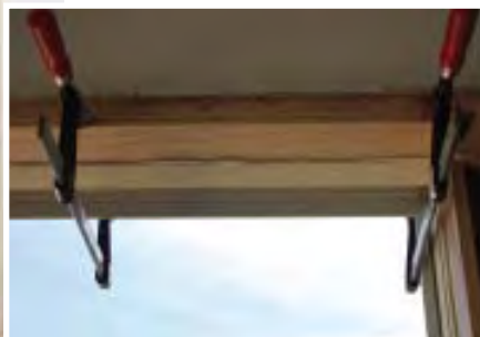
Figure 11. Here, the author applies a bead of fast-curing polyurethane glue to the edge of the extension jambs for a mullied window unit (above). Bar clamps squeeze the trim kit against the window jambs and plaster (left). The glue foams as it cures and the excess must be cut away while still pliable (below).
