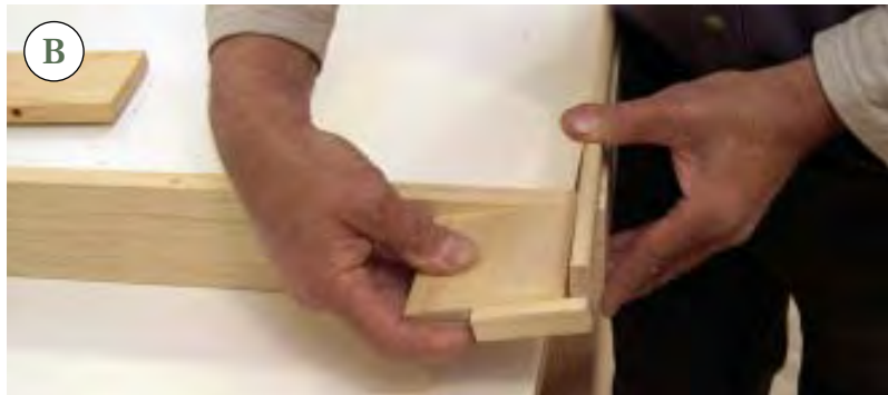
Figure 7. A spot of hot-melt adhesive (A) at either end of the parting bead groove provides fast installation of the bead, which — like the sill — has horns. A wood stop-gauge sets an accurate casing overhang for the parting bead (B). The author “tacks” and squares the sill to the jamb ends with two dots of hot-melt (C), then makes it permanent with a pair of countersunk drywall screws (D).
