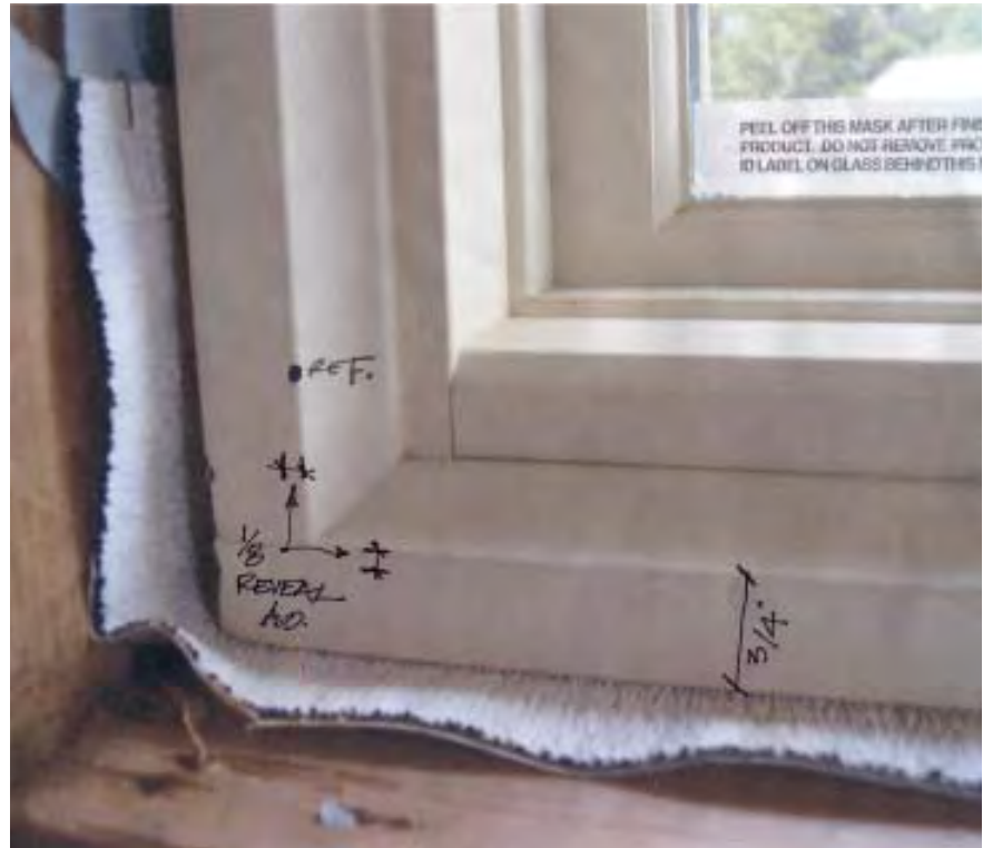
Figure 2. Digital photography provides a foolproof record of special site conditions. This printout has been marked up for concise shop reference.
