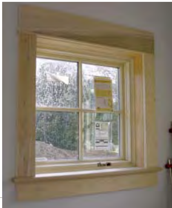
Figure 1. Window trim kits ship to the site in three pieces: the jamb extensions with sill, side casings, and parting bead attached; the head casing; and the apron.
