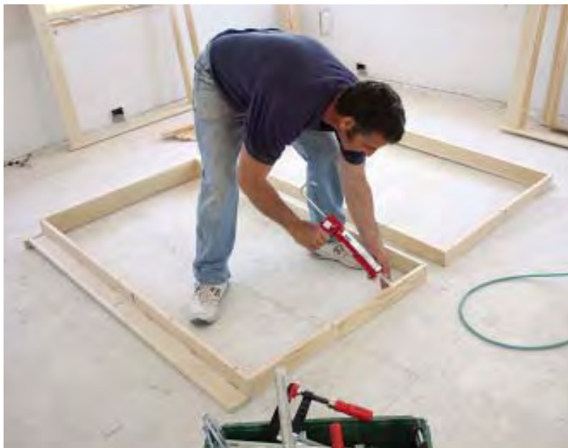
Figure 11. Here, the author applies a bead of fast-curing polyurethane glue to the edge of the extension jambs for a mullied window unit (above). Bar clamps squeeze the trim kit against the window jambs and plaster (left). The glue foams as it cures and the excess must be cut away while still pliable (below).
