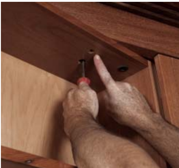
Figure 5. To install the case, the author first retracted the top pivot (top left), then rocked the case into place (above). At this point he realized he had forgotten to provide a screw-driver access hole to drop the pivot back into place. By trial and error he was able to drill a hole from underneath (left).
