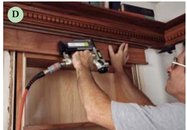
Figure 6. After swinging the case, the author attached the finish sides (A), then installed a shim made from high-density plastic to support the bookcase from beneath (B). With the case in its final closed position, he scribed and installed the bead (C) and head trim (D), leaving only a slight gap to allow the case to open.
