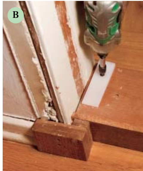
Figure 6. After swinging the case, the author attached the finish sides (A), then installed a shim made from high-density plastic to support the bookcase from beneath (B). With the case in its final closed position, he scribed and installed the bead (C) and head trim (D), leaving only a slight gap to allow the case to open.
