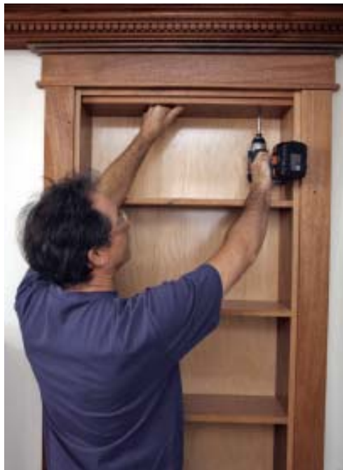
Figure 7. A mahogany dowel (far left) locks the closed book-case in place. A false top panel (left) completes the job.
