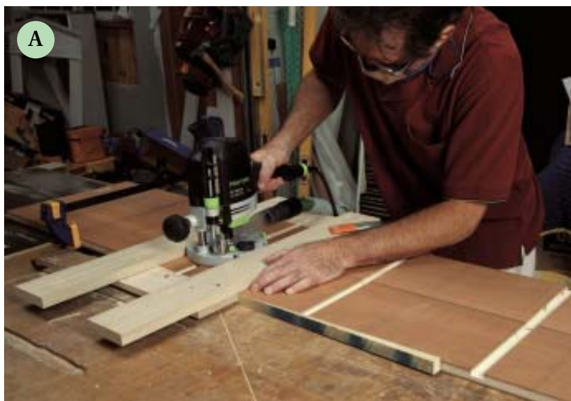
Figure 1. To strengthen the bookcase so it wouldn't sag, the author cut dados for the shelves (A). Before applying solid wood banding to the shelf edges, he ran them over a Collins Ply Prep bit (B), which helps achieve a tight glue line (C). The finished side on the strike side had to be beveled (D) to clear the jamb.
