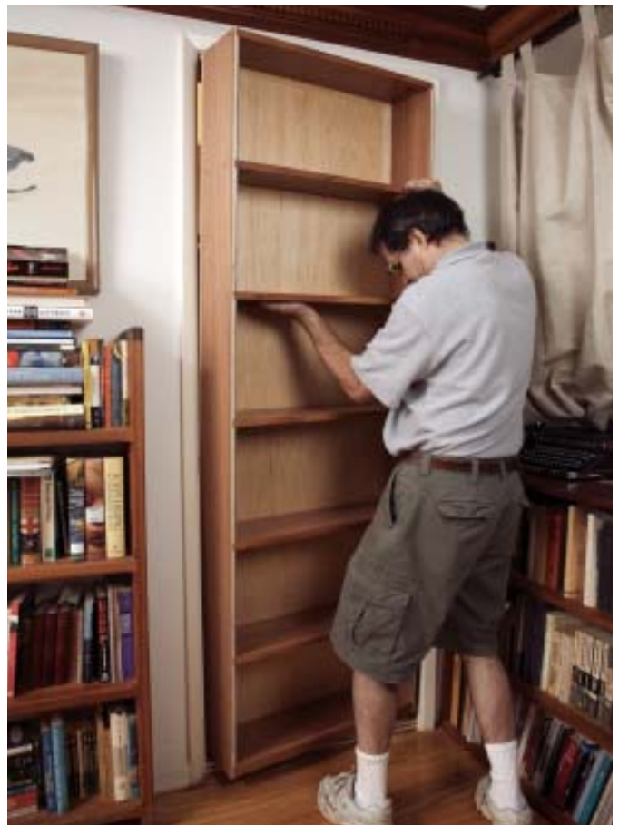
Figure 5. To install the case, the author first retracted the top pivot (top left), then rocked the case into place (above). At this point he realized he had forgotten to provide a screw-driver access hole to drop the pivot back into place. By trial and error he was able to drill a hole from underneath (left).
