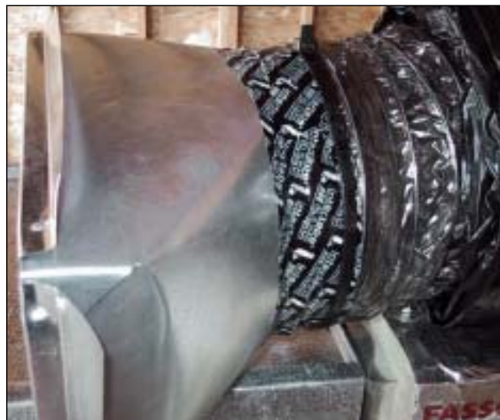
FIGURE 5. The photo on the left shows a poor (but unfortunately, common) duct connection to a boot. It should be executed as shown in the photo below: Peel back the cover and fix the liner to the boot with acrylic tape and a draw band, as shown. To complete the connection, pull the cover back down. Tape and secure this with a drawband as well.
