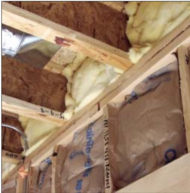
FIGURE 1. Fiberglass is not an air stop and cannot be relied upon to seal the rim joist (left). Best practice calls for sealing this area with spray foam (above).
