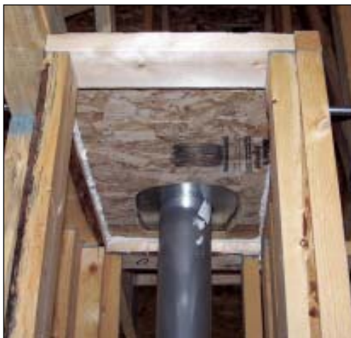
FIGURE 3. The top of a vent chase can dump a lot of conditioned air into an attic. Prior to installing the vent, cap the chase with OSB and seal the edges with a foam sealant, then seal the vent to the OSB with a metal collar.
