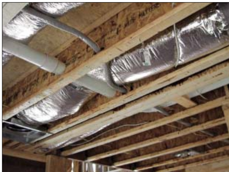
FIGURE 8. Coordinate the mechanical trades: This conflict between the HVAC duct and a plumbing drain could have been avoided by both trades meeting and reviewing the plans prior to the crews' arrival on site.
