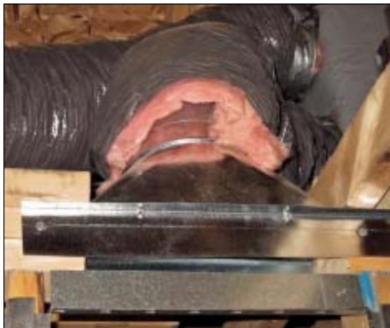
FIGURE 5. The photo on the left shows a poor (but unfortunately, common) duct connection to a boot. It should be executed as shown in the photo below: Peel back the cover and fix the liner to the boot with acrylic tape and a draw band, as shown. To complete the connection, pull the cover back down. Tape and secure this with a drawband as well.
