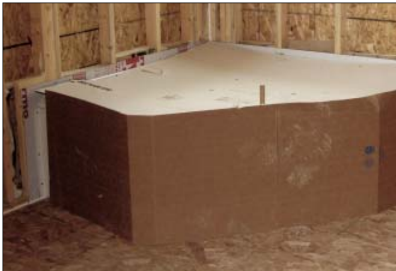
FIGURE 4. Before installing a tub unit, the wall cavity must be insulated and sheathed to stop the free transfer of air and energy. Thermo-ply or a similar type of sheathing is a good choice for this application because it doesn't pack the wall out too far.
