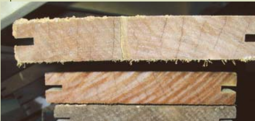
Figure 9. Tropical hardwood decking is fastened with the Eb-Ty connector system, which uses a slot-mounted plastic biscuit. Rather than cutting individual slots with a biscuit jointer, the author increases productivity by ordering deck boards with premilled grooves.
