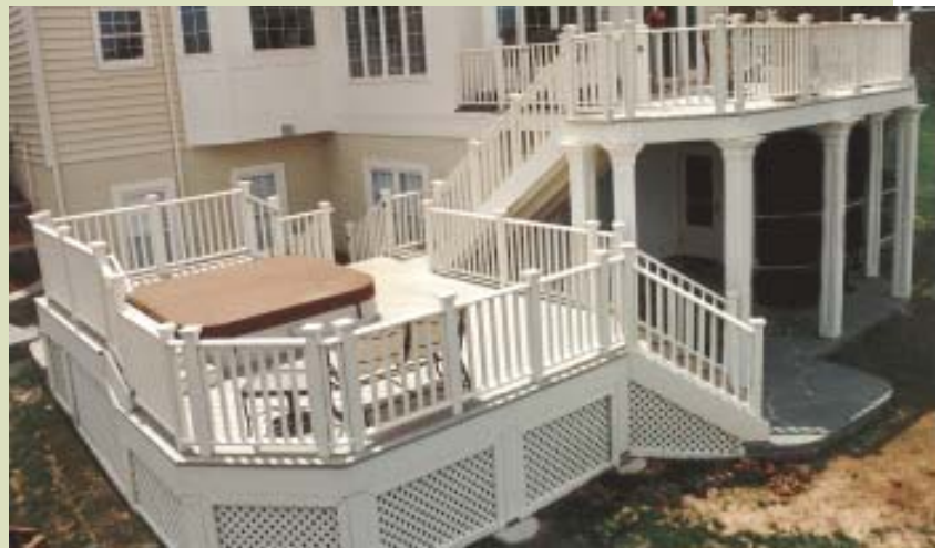
Figure 5. Enclosing the base of a deck with paneling or lattice provides a ground-hugging look and prevents it from appearing spindly. Where an elevated deck is located above a walkout basement, substantial support posts help provide a solid feel.
