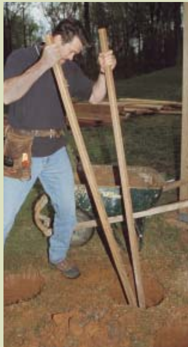
Figure 6. The basic frame of the deck is assembled on temporary posts placed where they won't interfere with the permanent posts (above). The site for each footing is determined with a plumb bob, and the holes are dug by hand (right). Once the concrete piers have been finished flush with the grade and drilled to accept an expansion bolt, the posts are fastened to post anchors with a palm nailer (far right).
