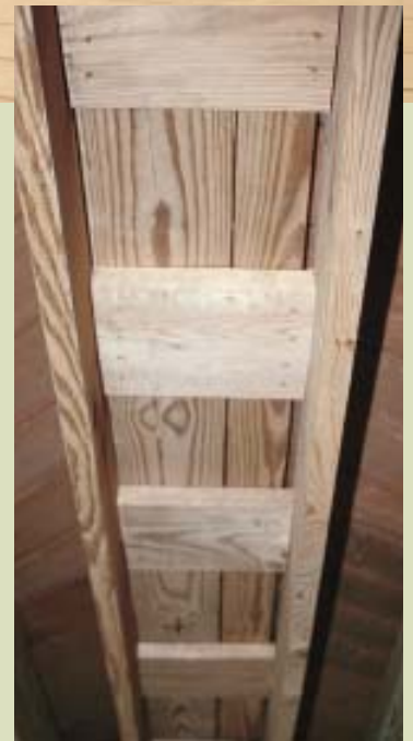
Figure 7. Running the deck boards diagonally eliminates unsightly butt joints. The layout is planned so that no individual board will be longer than 20 feet (top). Joists are spaced on 1-foot centers to provide a stiff surface underfoot. Where adjacent diagonal runs meet, an inlet strip, fastened to blocking between joists (above), provides a pleasing transition.
