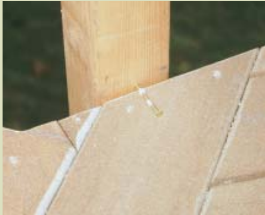
Figure 10. A “hanger nail” driven into a precut post at the level of the deck surface provides temporary support while the post is tack-nailed in place before bolting (above). To provide a simpler, stronger installation, posts are paired at either side of angle transitions and corners. The 4-inch gap between posts corresponds to the standard baluster spacing (right).
