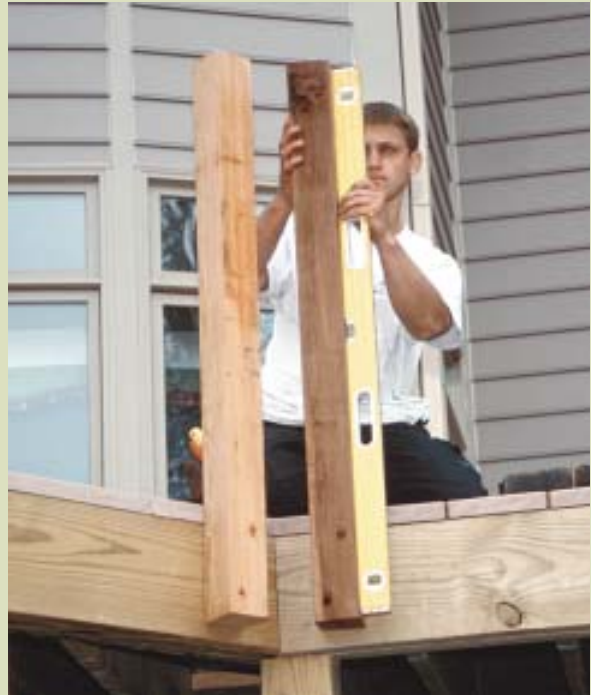
Figure 10. A “hanger nail” driven into a precut post at the level of the deck surface provides temporary support while the post is tack-nailed in place before bolting (above). To provide a simpler, stronger installation, posts are paired at either side of angle transitions and corners. The 4-inch gap between posts corresponds to the standard baluster spacing (right).
