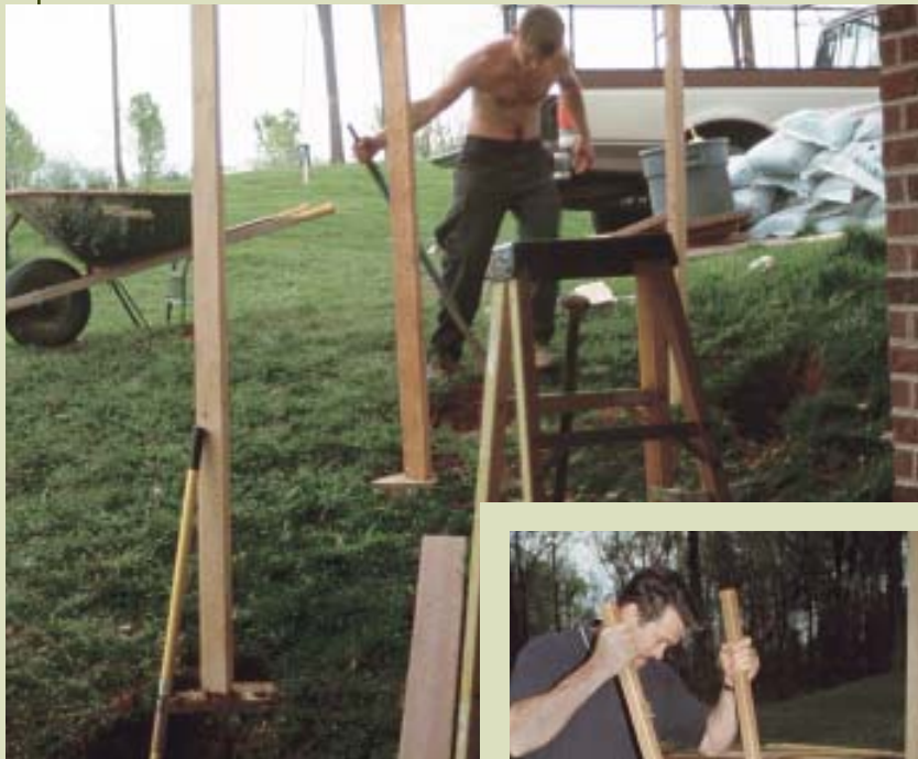
Figure 6. The basic frame of the deck is assembled on temporary posts placed where they won't interfere with the permanent posts (above). The site for each footing is determined with a plumb bob, and the holes are dug by hand (right). Once the concrete piers have been finished flush with the grade and drilled to accept an expansion bolt, the posts are fastened to post anchors with a palm nailer (far right).
