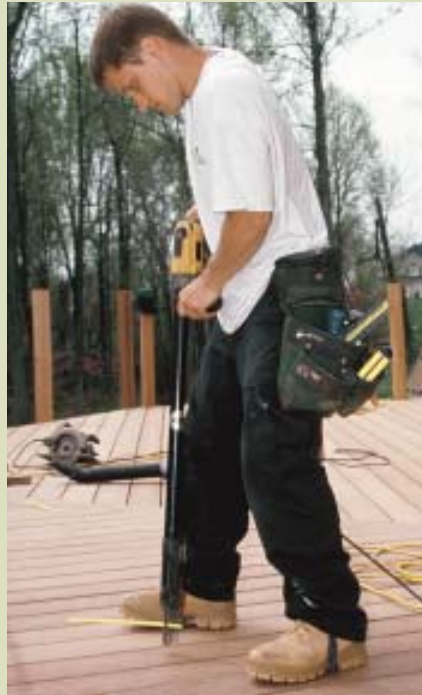
Figure 8. The decking is fastened with trim-head screws, which are buried slightly below the surface of the composite decking. Each screw creates a small “mushroom” that is hammered flat to conceal the screw head.
