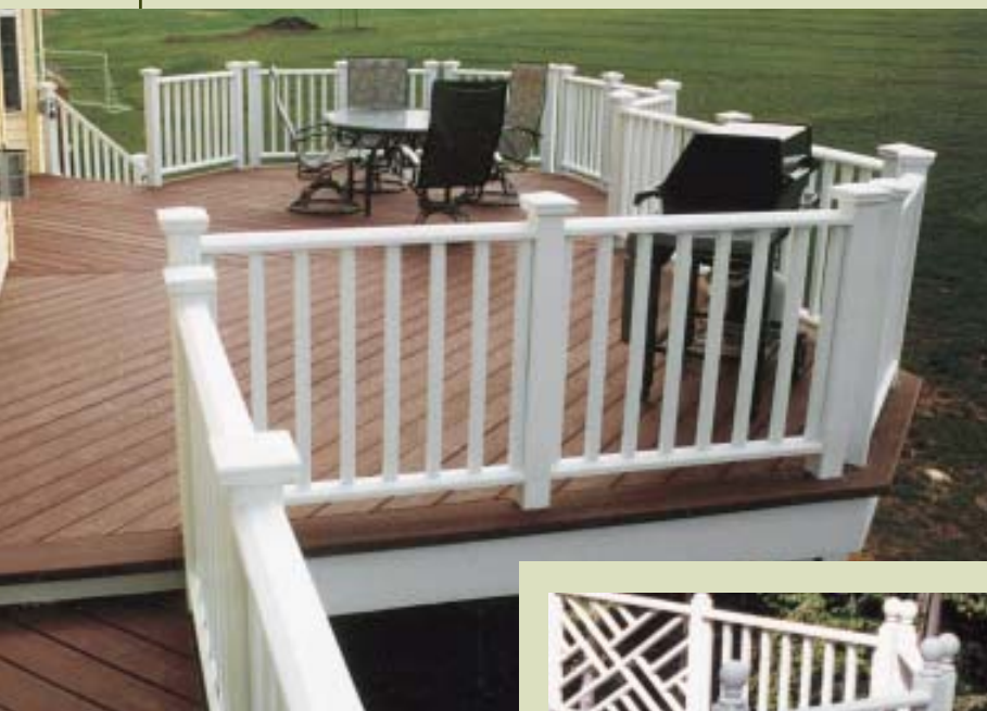
Figure 2. The author's base-priced deck uses a square-baluster-and-rail system, but a broad range of additional styles are available for a variable upcharge, which is calculated by the linear foot. The Madison Colonial (above) is a modest upgrade, while the ornate Chippendale railing (right) is a premium-priced option.
