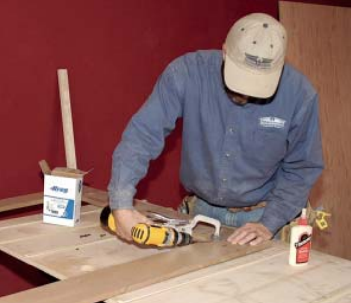
Figure 4. The author joins the MDF stiles and rails of the nine main ceiling panels with pocket screws (left), then pins the 1/4-inch birch plywood back in place, angling the nailer so the brads don't penetrate the face of the frame (right). The panels are trimmed with panel molding before being installed.
