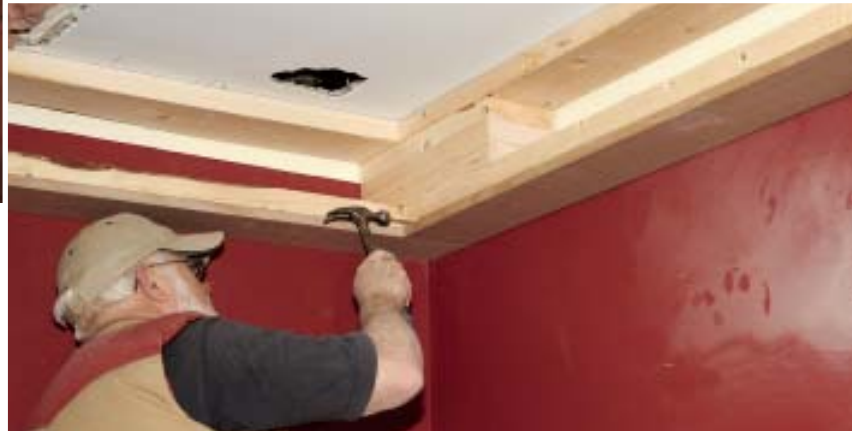
Figure 2. After snapping chalk lines for the major and minor beams, the author and his crew install 2-by blocking, using a square to help keep the top and bottom layers aligned. The beam bottoms are ripped from 16-foot lengths of MDF shelving and installed first. At the joints, shims are used to keep the bottom faces flush (right).
