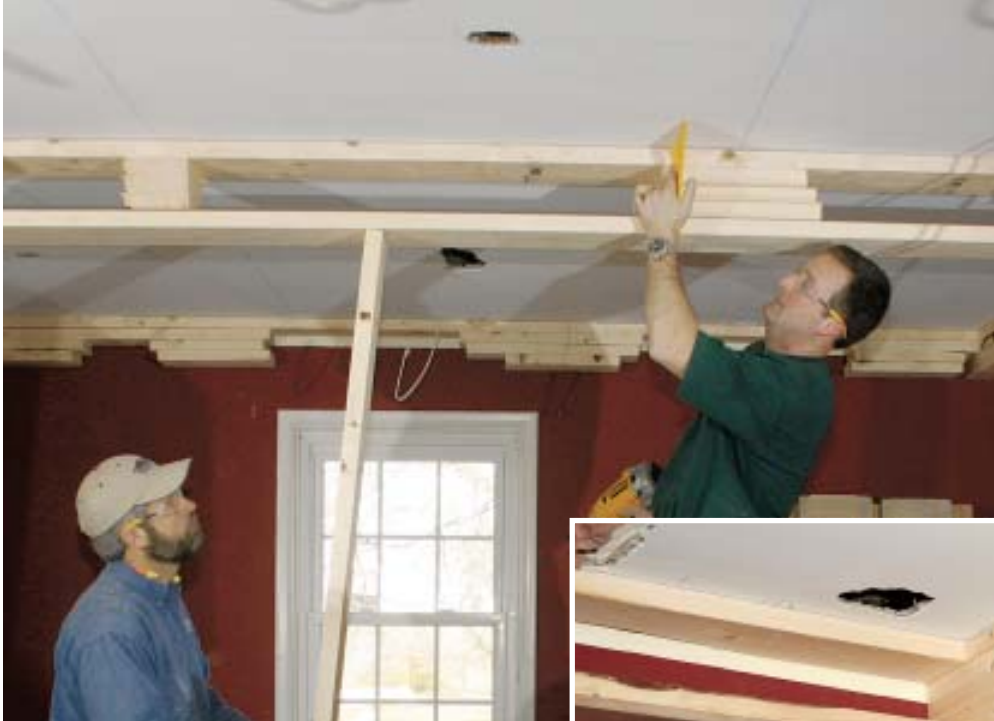
Figure 2. After snapping chalk lines for the major and minor beams, the author and his crew install 2-by blocking, using a square to help keep the top and bottom layers aligned. The beam bottoms are ripped from 16-foot lengths of MDF shelving and installed first. At the joints, shims are used to keep the bottom faces flush (right).
