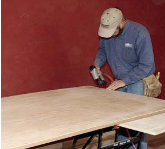
Figure 4. The author joins the MDF stiles and rails of the nine main ceiling panels with pocket screws (left), then pins the 1/4-inch birch plywood back in place, angling the nailer so the brads don't penetrate the face of the frame (right). The panels are trimmed with panel molding before being installed.
