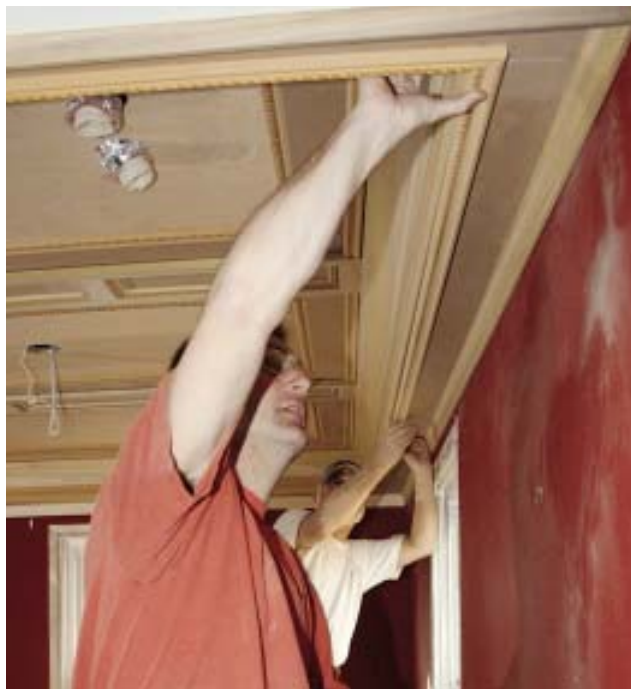
Figure 7. The final three moldings that finish the ceiling cover the filler strip above the crown molding, the joint where the bottom and edge of the beam meet, and the gap between the perimeter beam and the wall.
