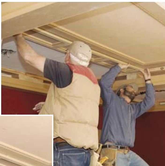
Figure 5. Guided by the snapped layout lines, the author installs the middle panel in each section first, using construction adhesive and nails to hold it in place (above left). A paneled minor beam overlaps the ceiling panels (above); it's temporarily fastened in place with a few nails along one edge only, allowing the next ceiling panel to be slipped into place underneath it. After making any necessary minor adjustments to the position of the panels, the author nails them off with a finish nailer (left).
