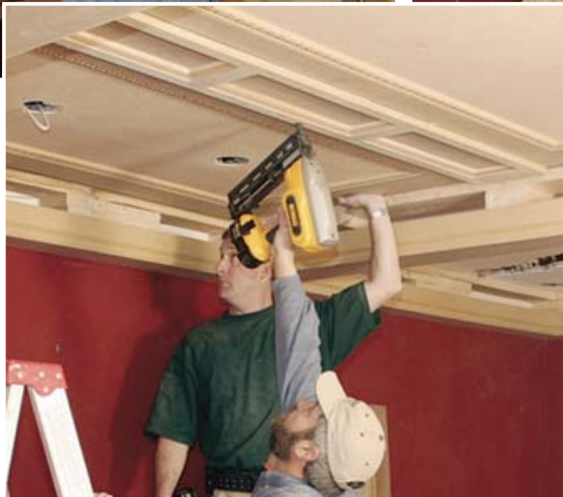
Figure 5. Guided by the snapped layout lines, the author installs the middle panel in each section first, using construction adhesive and nails to hold it in place (above left). A paneled minor beam overlaps the ceiling panels (above); it's temporarily fastened in place with a few nails along one edge only, allowing the next ceiling panel to be slipped into place underneath it. After making any necessary minor adjustments to the position of the panels, the author nails them off with a finish nailer (left).
