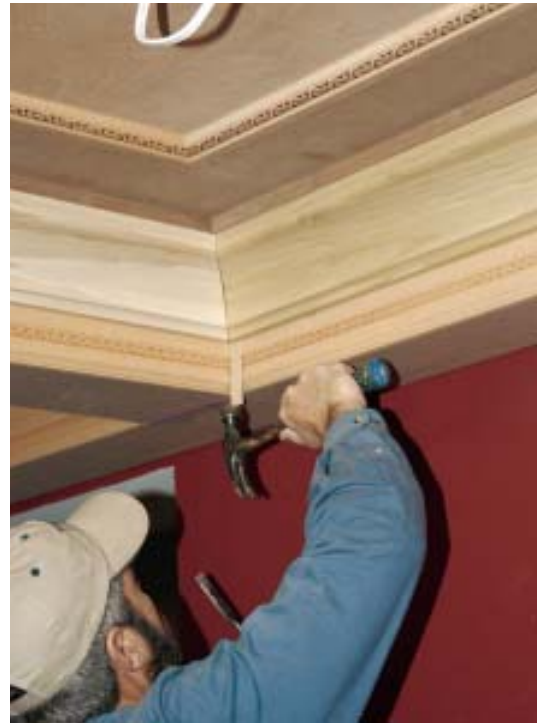
Figure 6. The crew uses spacer blocks to accurately mark the position of the filler strip and bottom edge of the crown molding (above). Instead of coping the corners, the author cuts the crown with inside miters, tapping in small shims to tighten up the joints where necessary (right).
