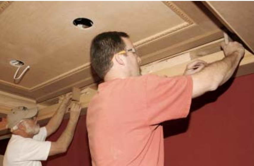
Figure 6. The crew uses spacer blocks to accurately mark the position of the filler strip and bottom edge of the crown molding (above). Instead of coping the corners, the author cuts the crown with inside miters, tapping in small shims to tighten up the joints where necessary (right).
