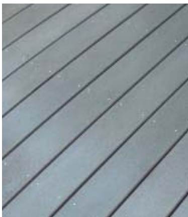
Figure 6. Yes, you can finish composite decking. No manufacturer requires that composite decking be finished, but colors can be changed, and older decks can be made to look newer.
