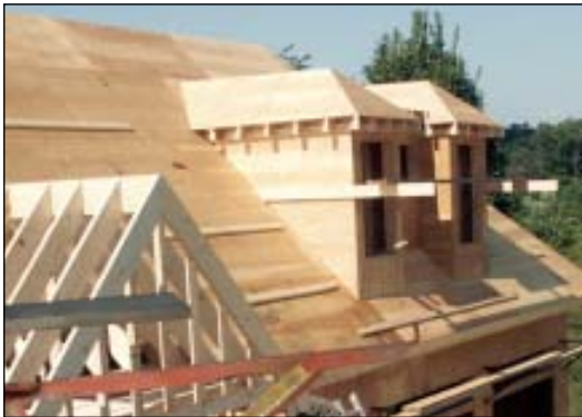
FIGURE 2. The trick to framing a Nantucket dormer is establishing the valleys for the two doghouse dormers (plan illustration above). The outside valleys meet the main roof, while the inside valleys meet the lower-pitched shed roof that joins the two doghouse dormers. While essentially a shed dormer in plan, the visual effect is closer to a pair of doghouse dormers (left).
