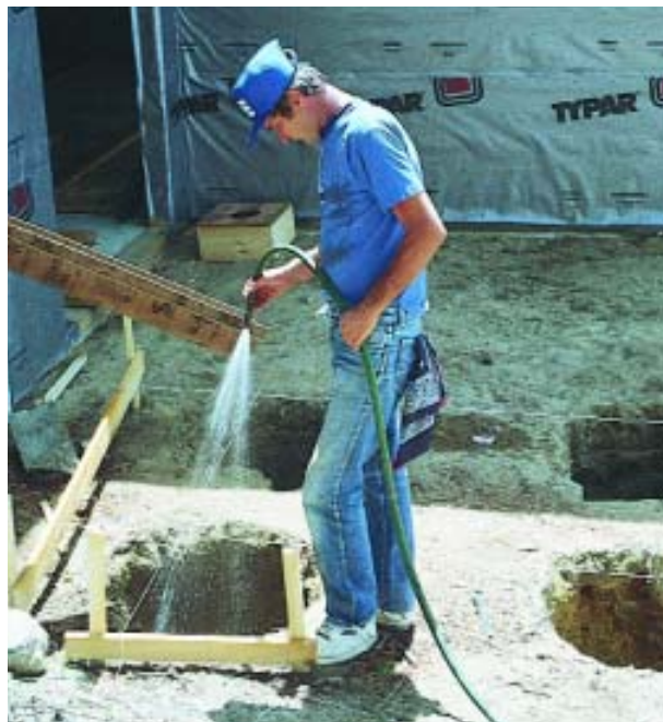
Figure 1. Saturating the pier hole with a garden hose helps compact the soil at the base to keep it from settling later.
