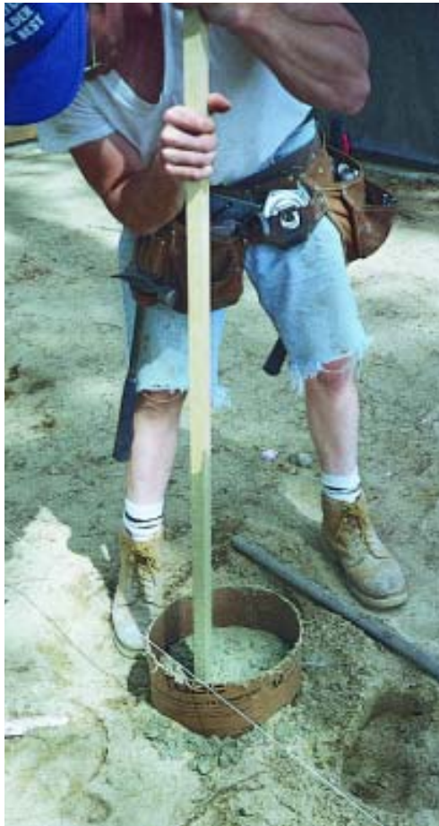
Figure 5. Tamping throughout the pour gets rid of voids in the pier. The nail in the side of the tube marks the finish concrete elevation.
