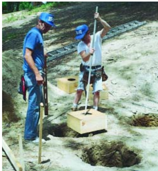
Figure 2. The author makes pier footing forms from scrap lumber and plywood, and lowers them into the hole with a hoe.
