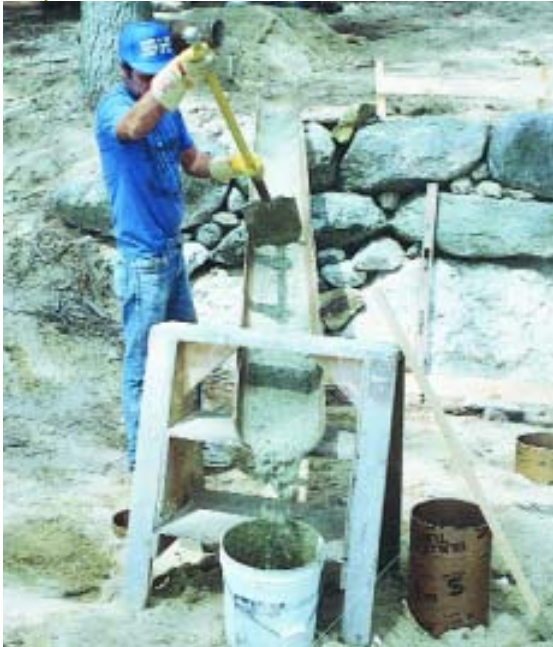
Figure 3. When mixing concrete by hand, a tube ripped in half with a circular saw makes a convenient chute (left).
