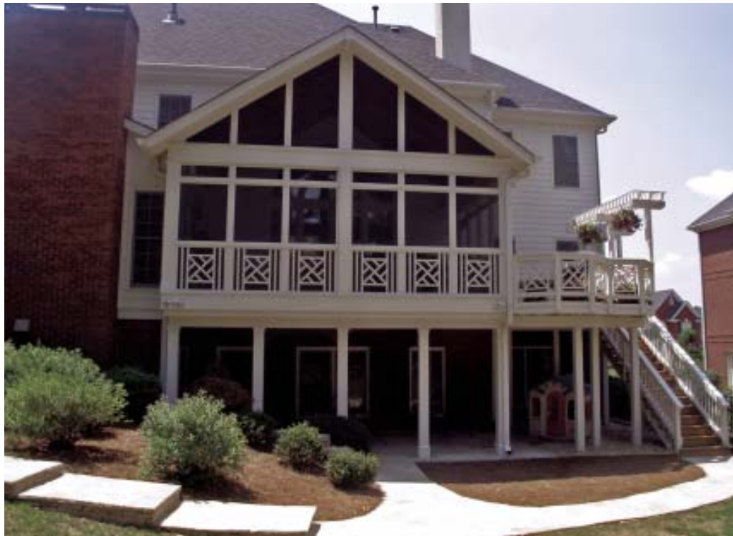
Figure 1. Elevated decks require more thought than ground-level decks. Difficulties of working at a height, safety concerns, increased footing loads, unfamiliar materials such as steel, and a greater need for lateral bracing all contribute to – and justify – significantly higher pricing.
