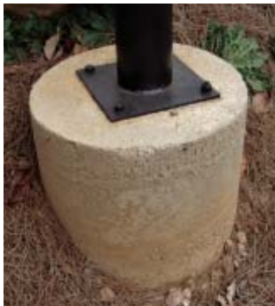
Figure 3. Piers rising above grade keep steel columns out of the dirt. Making them a larger diameter provides a larger target for locating the column, and helps to spread the load on the footing. Attaching columns with 1/2-inch bolts and wedge anchors adds stability and resists wind lift.
