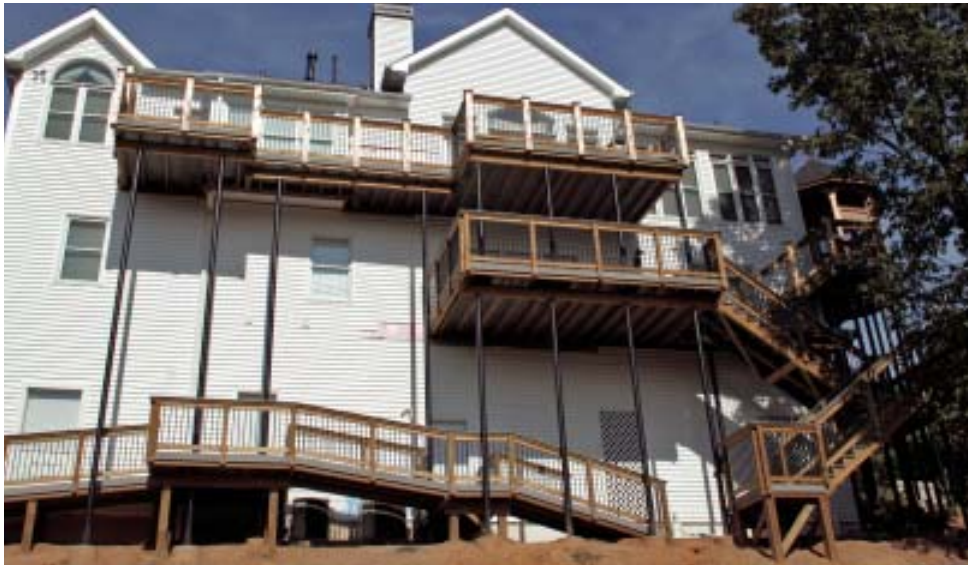
Figure 9. For decks elevated 13 or more feet, steel columns are needed to provide rigidity. Have the footings in place to determine column height before ordering.
