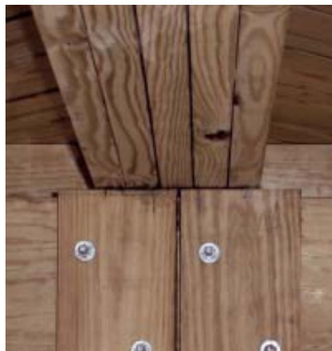
Figure 6. Multiple joists provide a continuous load path between upper-level and lower-level wood columns. Diagonally laid decking adds lateral stability.
