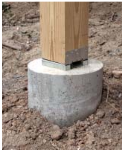
Figure 7. Using approved column bases takes on more importance on stacked decks. Be sure the ones used can handle the increased loads.
