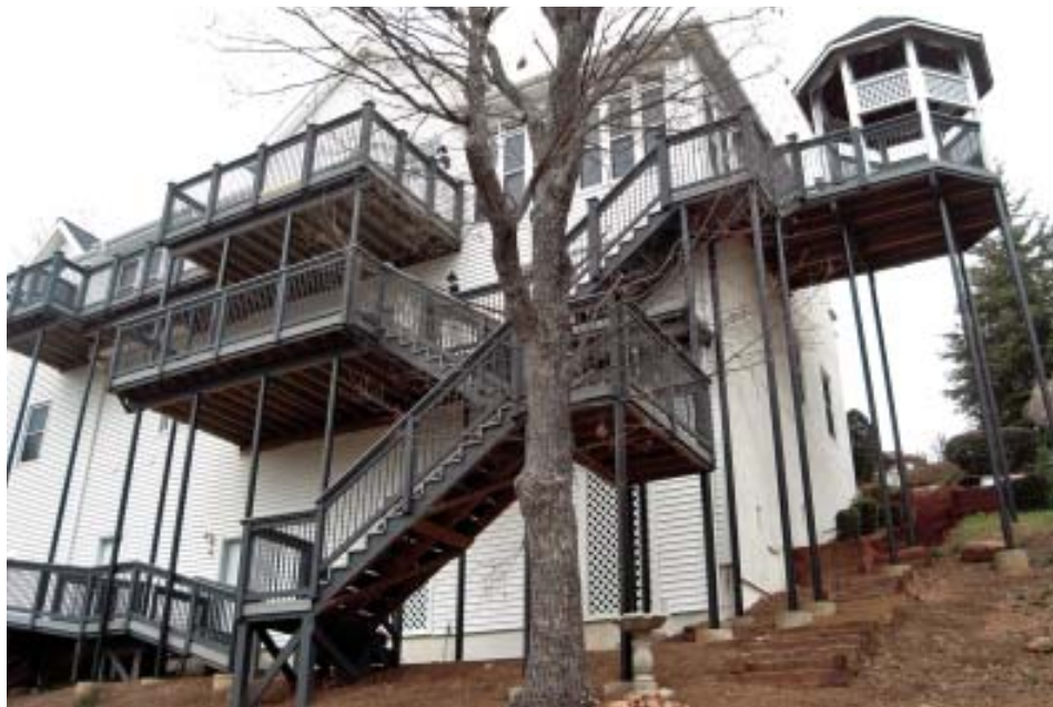
Figure 2. Bringing stairs off the end of the deck saves floor space. Very high decks require landings between levels. Having the stairs reach the ground close to the house, where the grade is highest, keeps them as short as possible.
