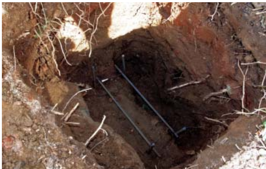
Figure 4. Footings for stacked decks need to be larger to support the increased loads. On sloping sites, special measures need to be taken to prevent the footing from sliding downhill; two such are digging a deeper footing, and digging the uphill side of the footing in deeper to provide a keyway.
