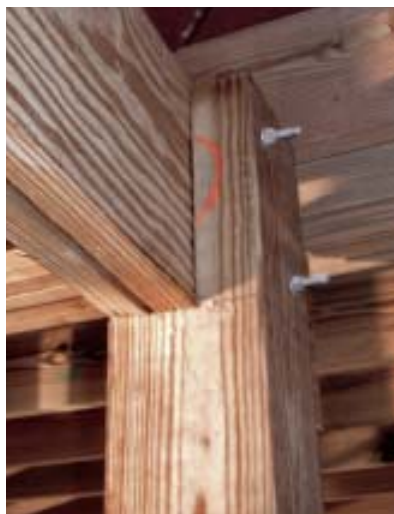
Figure 8. Notching 6x6 columns to receive a doubled 2-by beam provides a spot to positively anchor the beam to the column using bolts.
