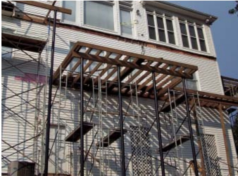
Figure 10. Bracing the beams on steel columns is done first with temporary 2x4s tied to the ledger, then more permanently using joists.
