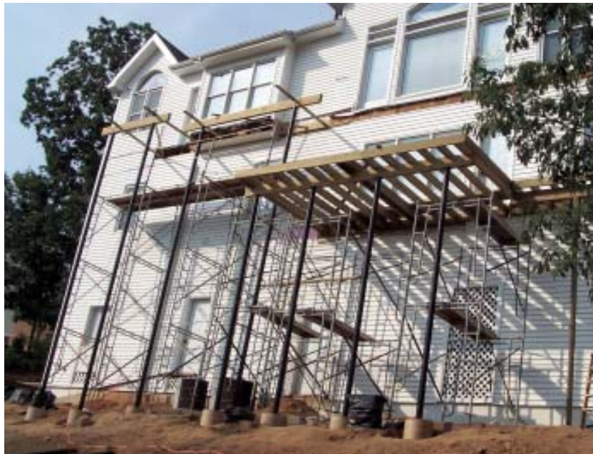
Figure 5. Scaffolding is essential to provide a safe and efficient workplace at a height. Be sure to rent enough to scaffold the sides and the width of the deck, and have extra walk boards to facilitate material handling.
