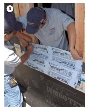
this 2x4 recess — I cut between the vertical and horizontal legs and fold the excess over the sides. For insets deeper than 6 inches, we extend the legs with a piece of peel-and-stick membrane placed underneath. We ensure that the corner flashing stays in place by stapling through the vertical legs. It's good policy to never staple through horizontal flashing (3, 4).
