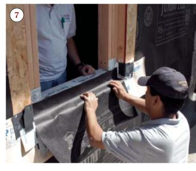
extra insurance (6), then install a piece of Grade D building paper over the peel-and-stick membrane to prevent UV damage and act as a slip sheet between the stucco and the flashing materials (7).
