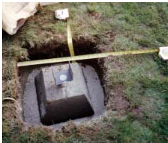
Figure 2. Washington's damp climate ensures that dry concrete mix placed below and around a footing pier has sufficient moisture to set up within one day.
