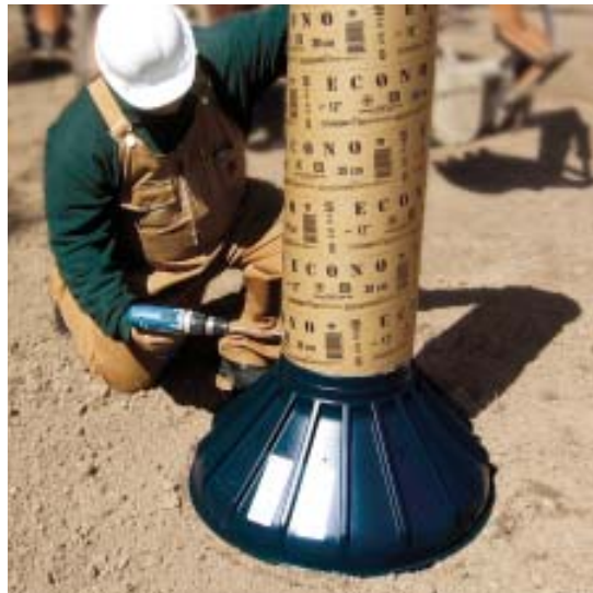
Figure 8. Footing forms attach to round form tubes to create a spread footing that can be backfilled and inspected prior to placing concrete.
