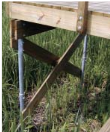
Figure 6. Like pin footings, helical footings are made from galvanized steel. No significant excavation is required for their installation, which can be done with a variety of machines with auger-driving capability.
