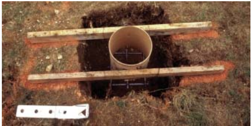
Figure 3. Framing lumber holds a footing-form tube above the bottom of the hole, allowing for a thickened spread footing. Backfilling is done after placing the concrete.
