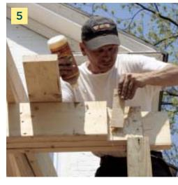
To support the porch roof, we attached a ledger to the solid brick building with a combination of 3/8-inch lags and lead shields and epoxied threaded rod (1). At the eaves, we used three-layer built-up 2x8 beams for the straight runs and a laminated beam for the radius, all supported by fiber-reinforced synthetic columns.
