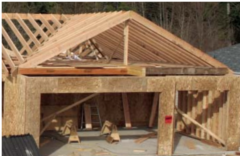
Figure 1. Framing a Dutch hip starts with the gable, which in this case sits 3 feet back from the end wall. The author uses 10\frac{3}{4} inches as the heel stand, or height-above-plate (HAP), because it provides adequate bearing at the rafter seat cuts of all three pitches that will form the corner. Given the HAP, the span, and the pitch, a Construction Master calculator makes it easy to find the rafter dimensions and the height of the center post. Note that the ridge beam is dropped 1 inch to allow for ventilation.
