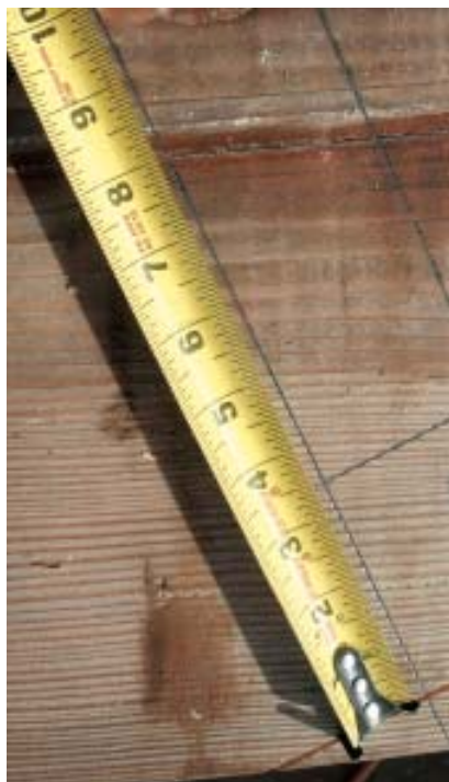
Figure 5. To speed construction, the author typically backs only one side of the hip. Starting from the top edge of the shallow-pitch side, he first measures down the birdsmouth heel cut line the HAP distance (far left). He then makes the seat cut through to the other side, flips the hip stock over, hooks his tape in the kerf, and measures back up the opposite heel cut line the same distance (left). This marks the line along which the steep side of the hip planes into the roof surface. A two-step process with a Construction Master calculator gives the backing angle (illustration). Note that the backing bevel does not reach the center of the hip; the other edge of the hip — still square — is set flush with the shallow-side rafters (below).
