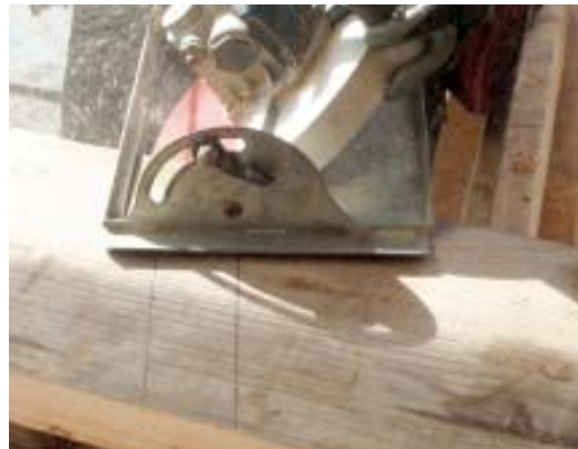
Figure 4. Before cutting the irregular hip rafter to length, the top and bottom plumb marks and the birdsmouth heel cut line must all be shortened, or set back, so that the bevel cuts meet at the hip centerline (below).
