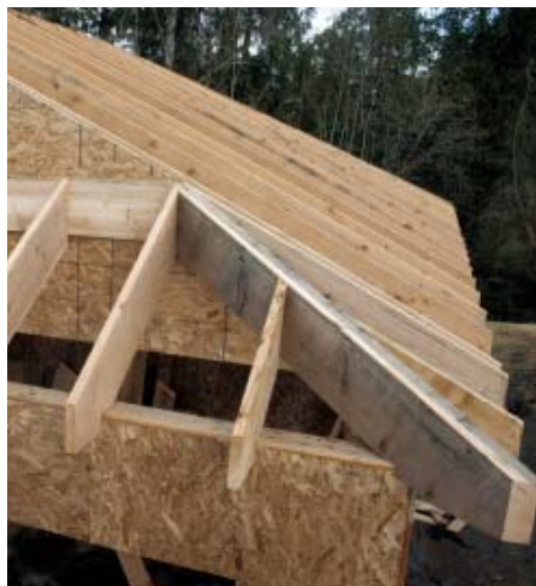
Figure 5. To speed construction, the author typically backs only one side of the hip. Starting from the top edge of the shallow-pitch side, he first measures down the birdsmouth heel cut line the HAP distance (far left). He then makes the seat cut through to the other side, flips the hip stock over, hooks his tape in the kerf, and measures back up the opposite heel cut line the same distance (left). This marks the line along which the steep side of the hip planes into the roof surface. A two-step process with a Construction Master calculator gives the backing angle (illustration). Note that the backing bevel does not reach the center of the hip; the other edge of the hip — still square — is set flush with the shallow-side rafters (below).
