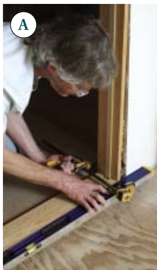
Figure 3. After the jamb is placed inside the rough opening, a spreader keeps the bottom square with the top, while a straightedge ensures that the assembly stays in plane with the wall (A). With the jamb centered in the rough opening, the bottom hinge is shimmed and tacked, with nails driven beneath the shims to permit adjustment (B). Then the top hinge gets the same treatment (C). Note that although the author is using a prehung door jamb in this photo sequence, installation of a site-assembled jamb set is exactly the same.
