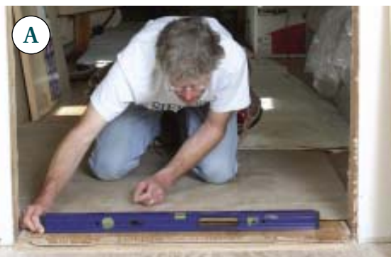
Figure 2. Before putting in the door jamb, the author checks the floor with a level to determine whether one side is higher than the other (A). Since this jamb is resting on top of finished flooring, the high side must be scribed (B) and trimmed, or the head jamb won't sit level. A fine-toothed Japanese pull saw is more accurate than a power saw and cuts almost as quickly (C).
