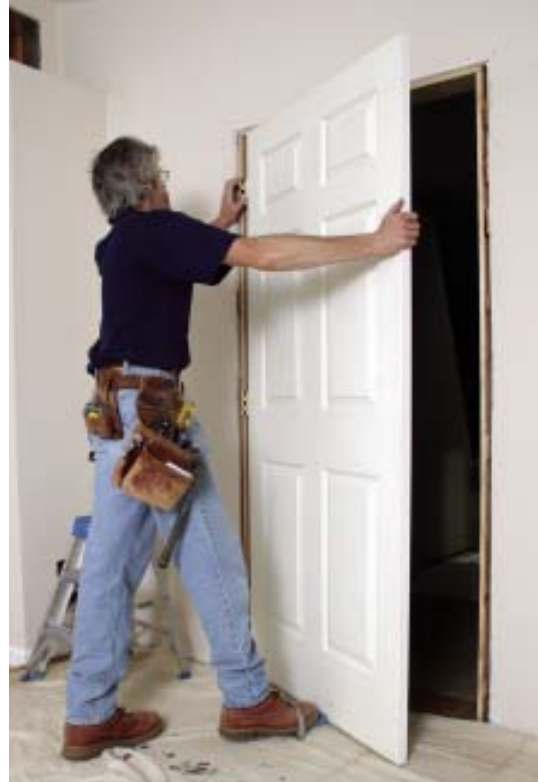
Figure 7. Although it's designed for drywall, a board lifter is an ideal tool for finessing a solid-core door onto its hinges. Unlike a pry bar, this tool has a built-in fulcrum as well as a stirrup, so you never need a third hand to reach down and reposition it.
