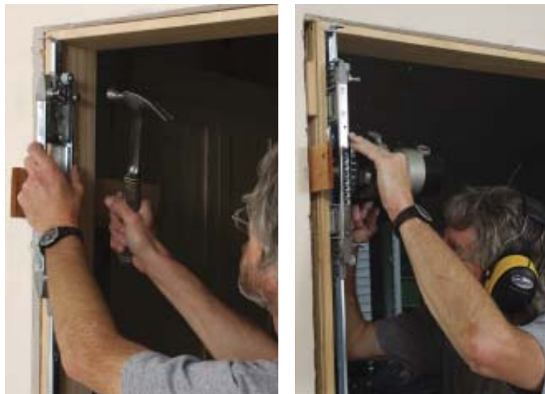
Figure 6. To cut the hinge mortises for the jamb, the author butts the template's end stop gauge tight to the head jamb, then makes sure before he sets the pins that the two thickness stops on either side of each hinge section are tight to the frame (above, left). He follows the same procedure for cutting the mortises as for cutting the door (above, right).
