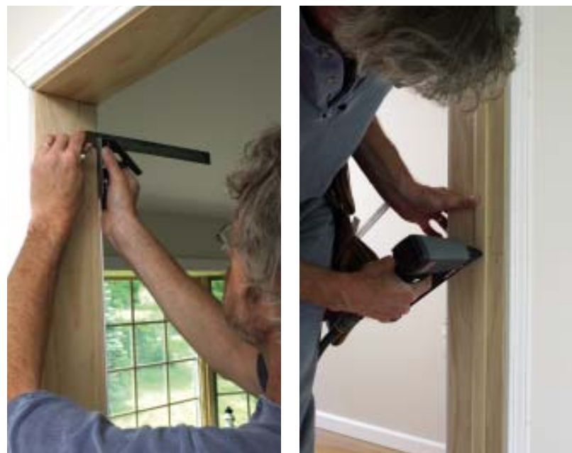
Figure 8. When it's time for door stops, the author scribes a pencil line the same thickness as the door on the face of the jamb (above, left). To prevent the door from binding, he leaves the line showing, except for at the point where the strike plate will go (above, right).
