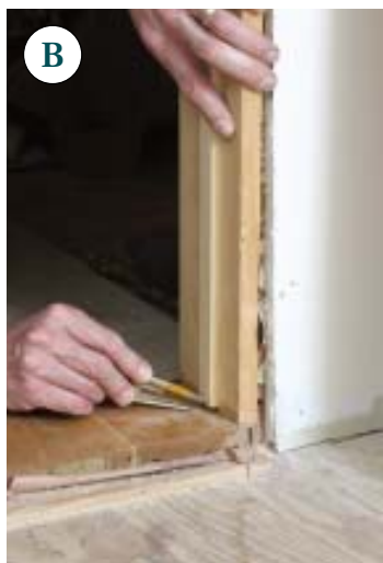
Figure 2. Before putting in the door jamb, the author checks the floor with a level to determine whether one side is higher than the other (A). Since this jamb is resting on top of finished flooring, the high side must be scribed (B) and trimmed, or the head jamb won't sit level. A fine-toothed Japanese pull saw is more accurate than a power saw and cuts almost as quickly (C).
