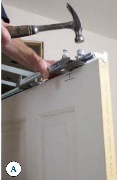
Figure 5. Before setting the pins that fasten a hinge mortising template, the author makes sure that the stops underneath and at the top fit tightly against the door (A). To work with a template, he fits the router with a 1/2-inch mortising bit encircled by a 5/8-inch template guide (B). This setup leaves rounded corners that are easily squared up with a soft tap on a corner chisel (C). A self-centering Vix bit ensures that the hinge screws lay flat (D).
