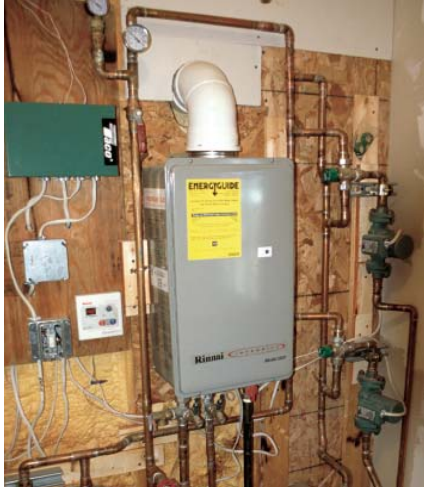
Figure 1. The compact Rinnai heater, pumps, mixing valves, and controls fit neatly on a utility-room wall. The wall-mounted box to the left of the unit is an LCD temperature adjustment control that lets the user match the heater's output to the needs of the house.
