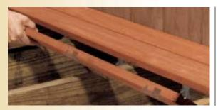
Working from above with the deck board upside down, you screw two polycarbonate IQ clips to the bottom of the board, centered approximately over each joist. You then flip the board over, and the inboard clip interlocks with the one on the previously installed board. The outboard clip is screwed to the top of the joist.
