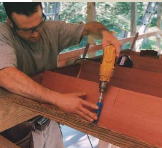
Figure 7. Using a Kreg jig, the carpenter drills three pocket screw holes into the top of the riser, then uses ACQ-rated 1 5 / 8 -inch deck screws to pull the tread and riser together (left). Next he predrills (above) before driving 2 1 / 2 -inch stainless steel screws through each riser into the back of the tread below.
