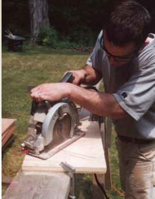
Figure 2. Because the site-built jig will guide the router, it's important to cut the template carefully. Here, a carpenter makes the first plunge cuts with a circular saw (left) and then finishes up with a jigsaw (above).
