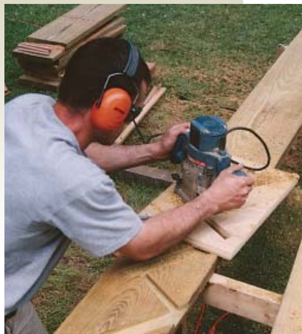
Figure 3. Using a plunge router with a \frac{3}{4} -inch-diameter pattern routing bit, the carpenter cuts \frac{1}{2} -inch-deep mortises in two passes. The jig is clamped to the stringer so that the top of the tread and the front of the riser align with the layout marks.
