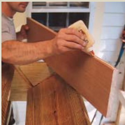
Figure 6. To set a riser, the carpenter runs a bead of glue along its top, then seats it in its mortises so that it contacts the tread above and smears the glue around, which helps prevent drips (right). Then he runs a bead of glue along the back of the tread before driving home wedges on each side of the riser (below).
