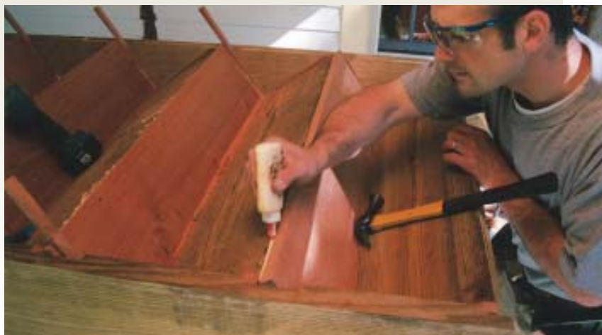
Figure 6. To set a riser, the carpenter runs a bead of glue along its top, then seats it in its mortises so that it contacts the tread above and smears the glue around, which helps prevent drips (right). Then he runs a bead of glue along the back of the tread before driving home wedges on each side of the riser (below).
