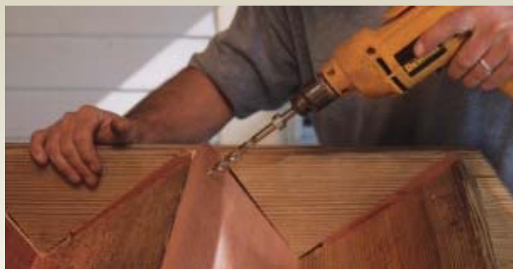
Figure 7. Using a Kreg jig, the carpenter drills three pocket screw holes into the top of the riser, then uses ACQ-rated 1 5 / 8 -inch deck screws to pull the tread and riser together (left). Next he predrills (above) before driving 2 1 / 2 -inch stainless steel screws through each riser into the back of the tread below.
