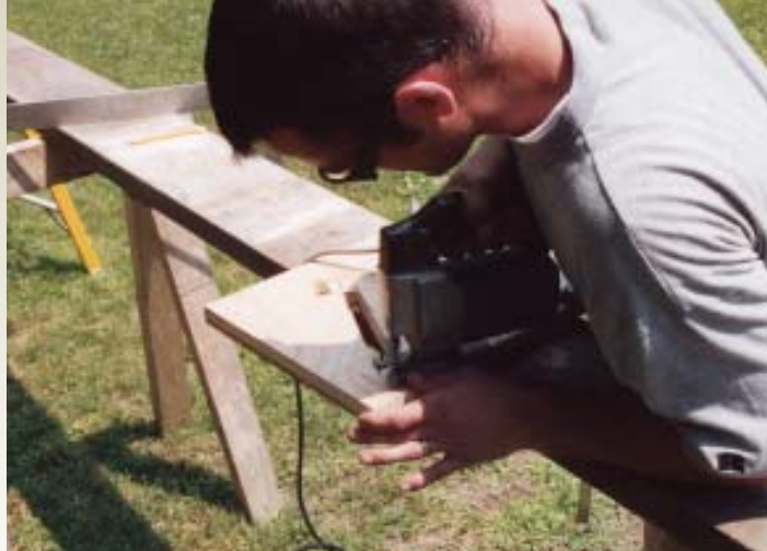
Figure 2. Because the site-built jig will guide the router, it's important to cut the template carefully. Here, a carpenter makes the first plunge cuts with a circular saw (left) and then finishes up with a jigsaw (above).
