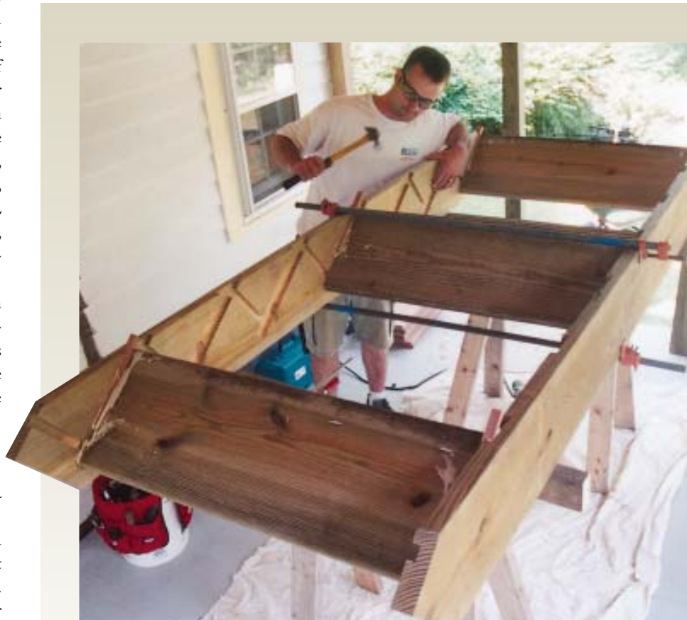
Figure 5. With the tread seated and the stringers bar-clamped together, the carpenter drives home a heavily glued wedge on each side.
